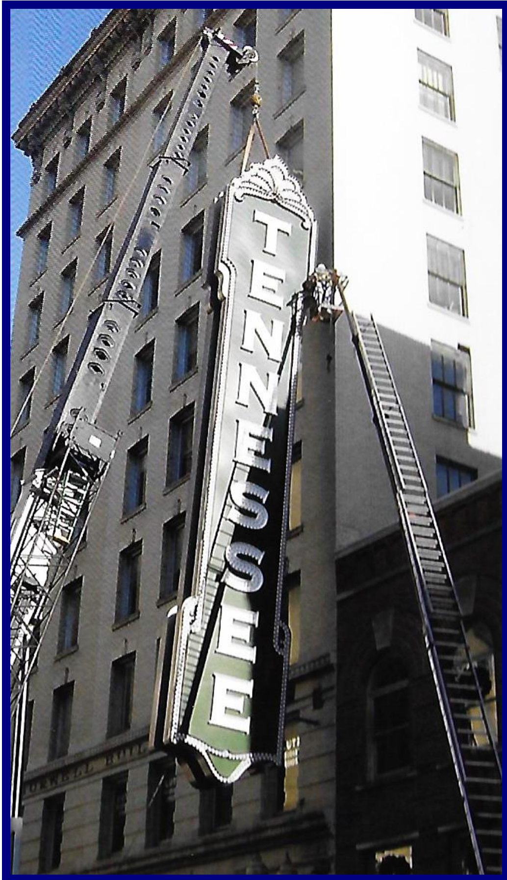
A new vertical sign being installed in December 2004.
