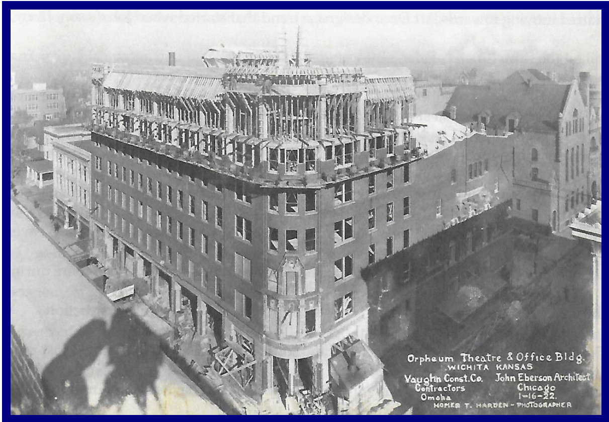
The Orpheum under construction in 1922. It opened the same year. The architect, John Eberson, pioneered "atmospheric" theatres, where the auditorium ceiling resembled the starlit night sky.
