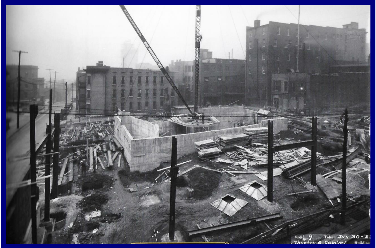
Construction underway in June 1928.
