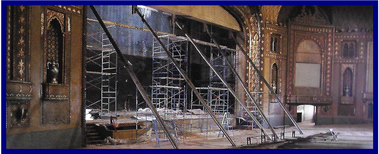
Support beams in the auditorium at the start of the 2003 renovations.
