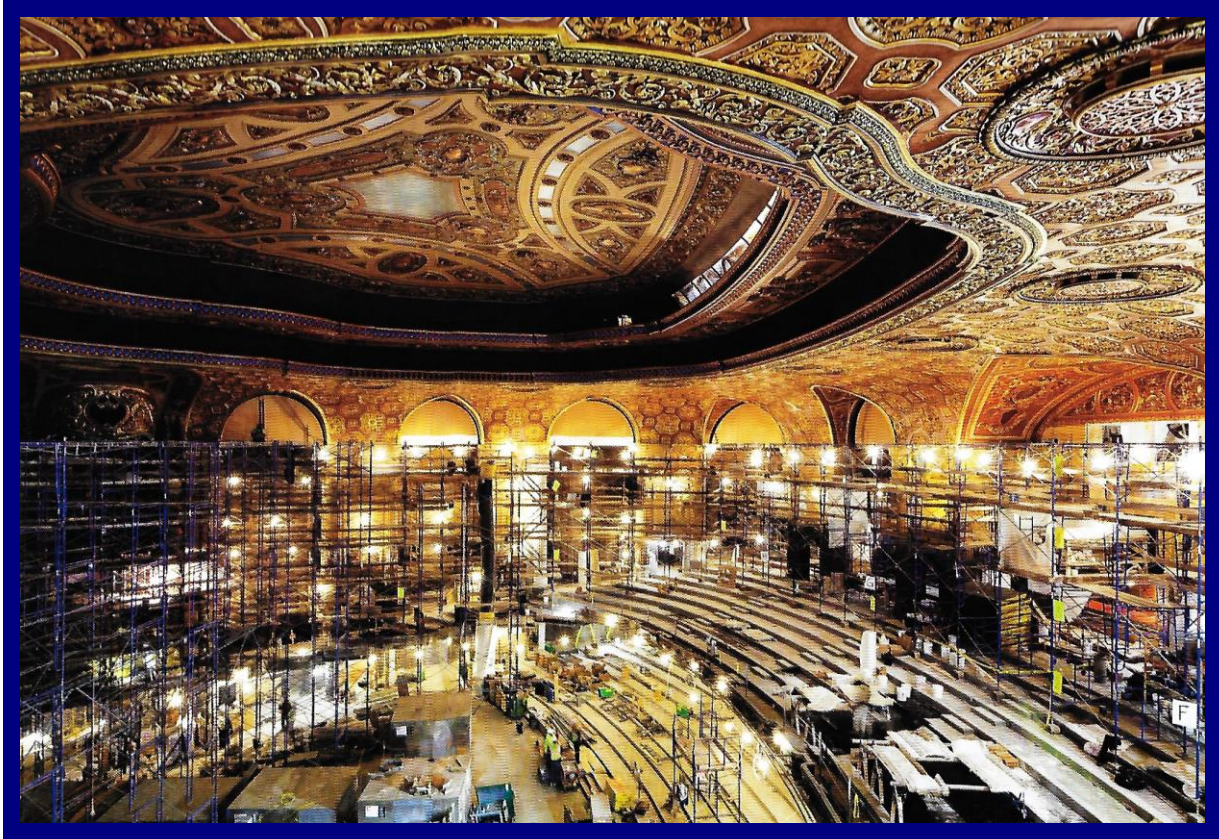
"Rebirth of the Kings": the complicated scaffolding in the auditorium.
