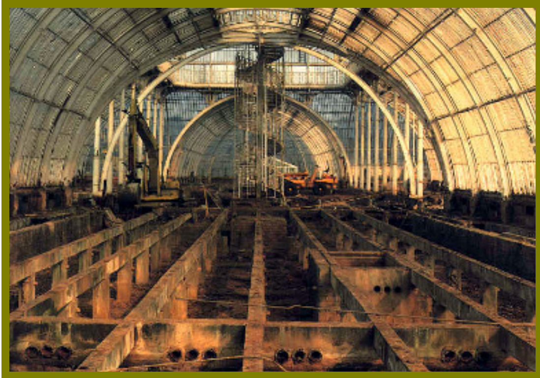
Restoration of Kew Palm House 1985. Underfloor heating pipes removed.
