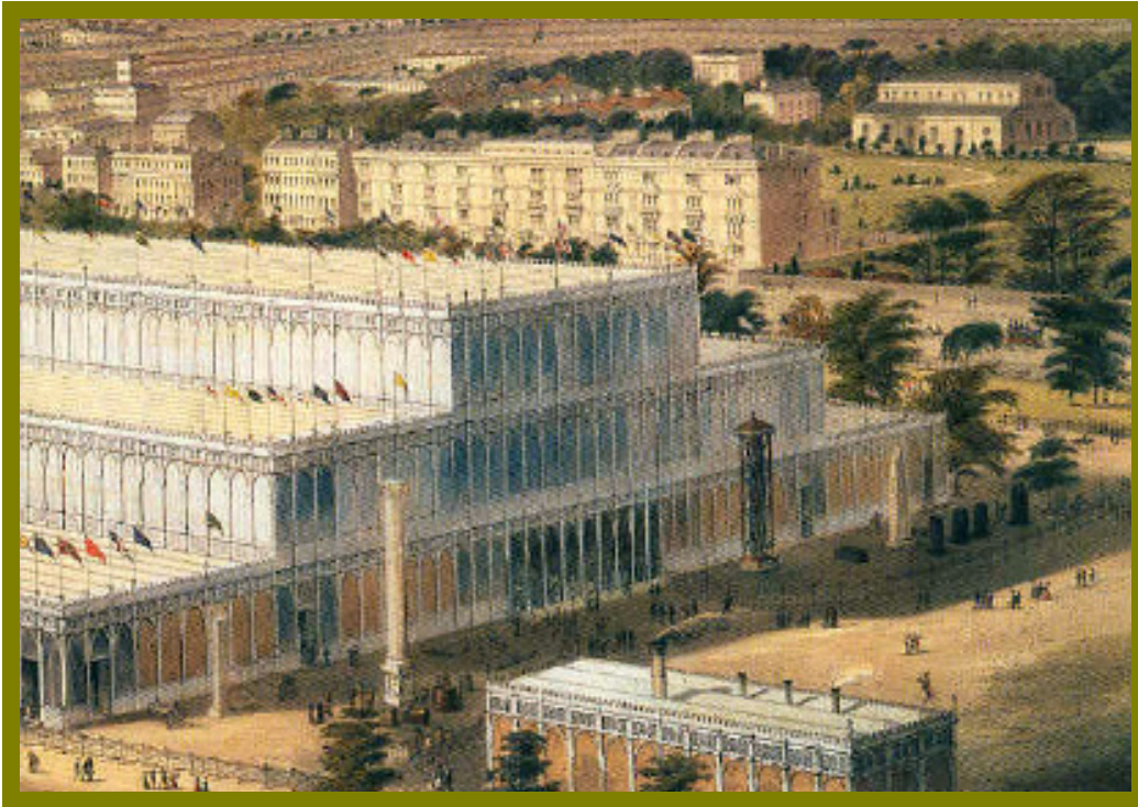
The boilerhouse (foreground) which generated steam to power the exhibits in the Machinery Hall of the Great International Exhibition. The Crystal Palace of 1851 in Hyde Park was a temporary structure and unheated.
