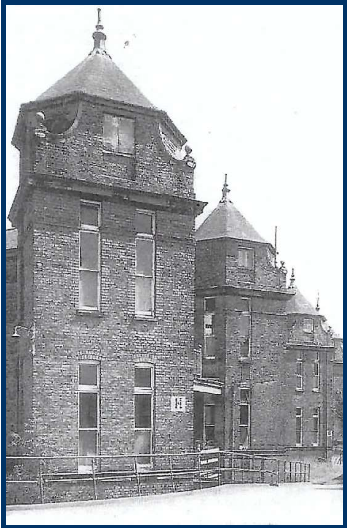
View of sanitary towers at the ends of the Ward Pavilions, 1897.
