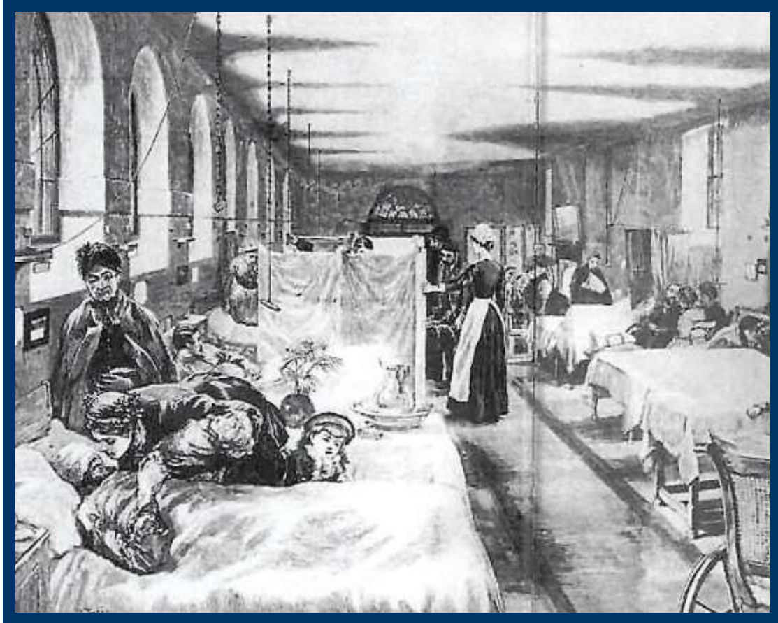
Visiting time in the Accident Ward: heated by open fireplace (far end, right-hand wall).
