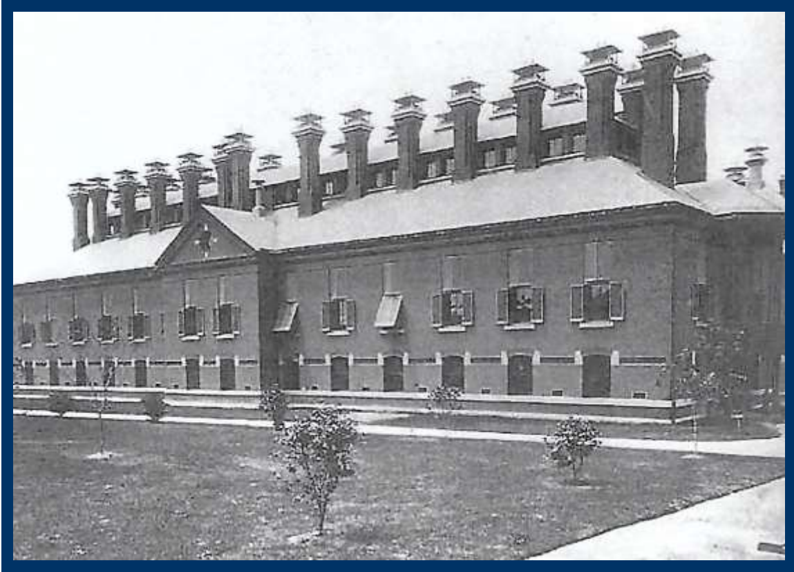
The Isolating Ward block, each patient having a separate room with its own ventilating system, the foul air being exhausted through the ranks of aspirating chimneys .
