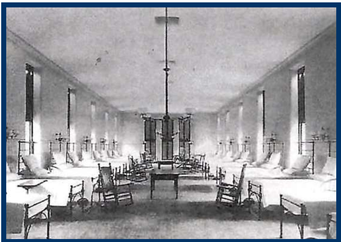
Common Ward with iron blacksmith beds, each having supply air outlet under c.1885
