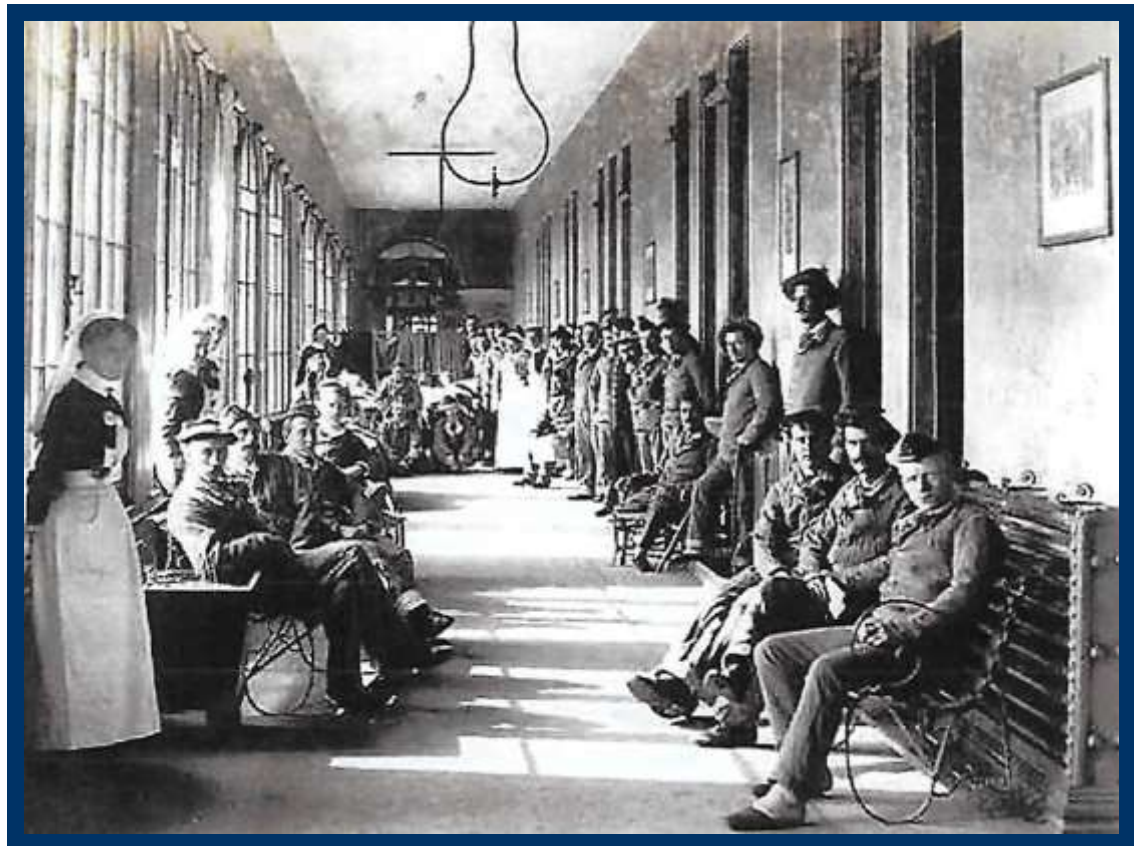
Military Hospital with patients from the Boer War: Box-End tubular radiator (right foreground).
