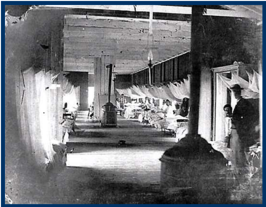
Harewood Army Hospital, solid-fuel stoves and kerosene lamp lighting.
