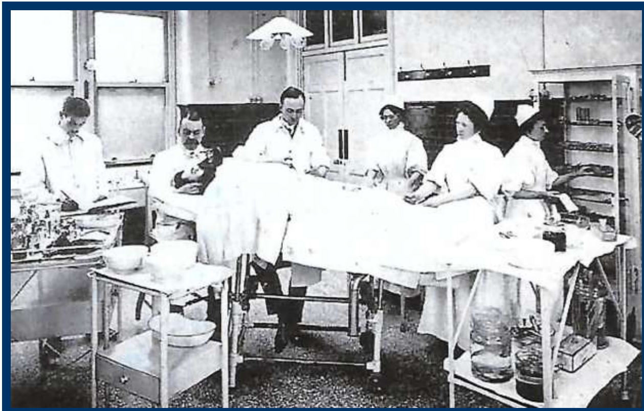
No heating visible. Opening sash windows. Staff wearing neither masks nor gloves.
