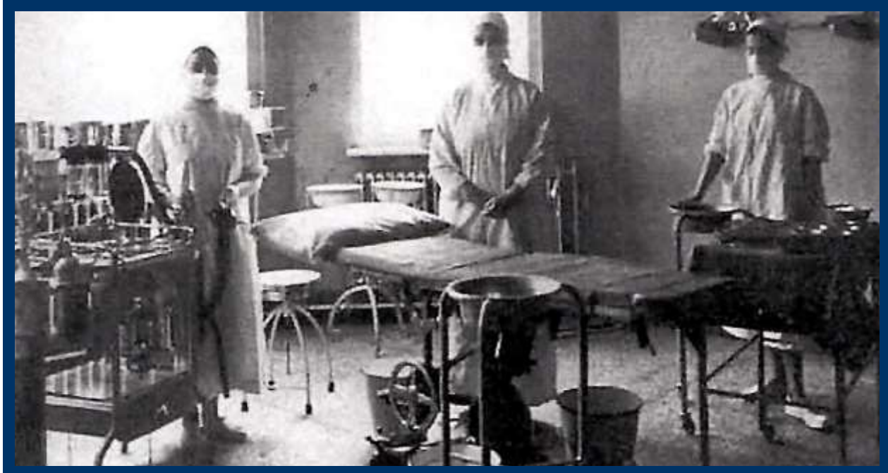
War Memorial Hospital c.1923 with 8 beds in 2 Public Wards. Radiator under window and (on left) trolley with medical gases.
