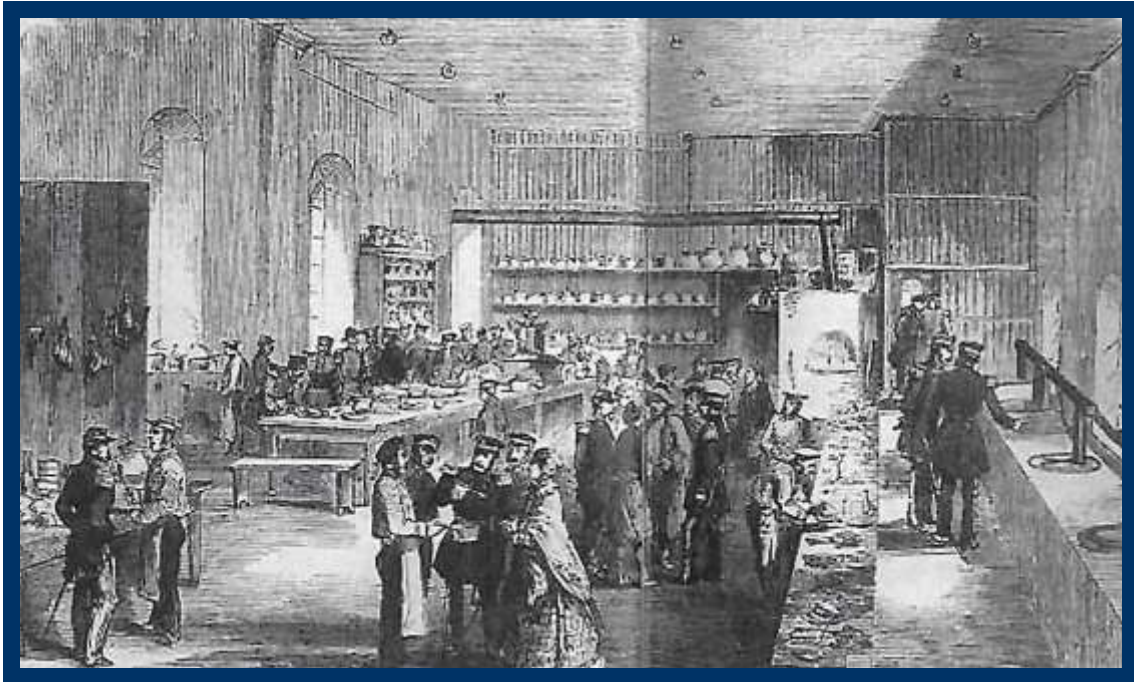
Kitchen of Alexis Soyer (previously chef at London's Reform Club) with boiler and a solid-fuel cooker, both with horizontal flues.
