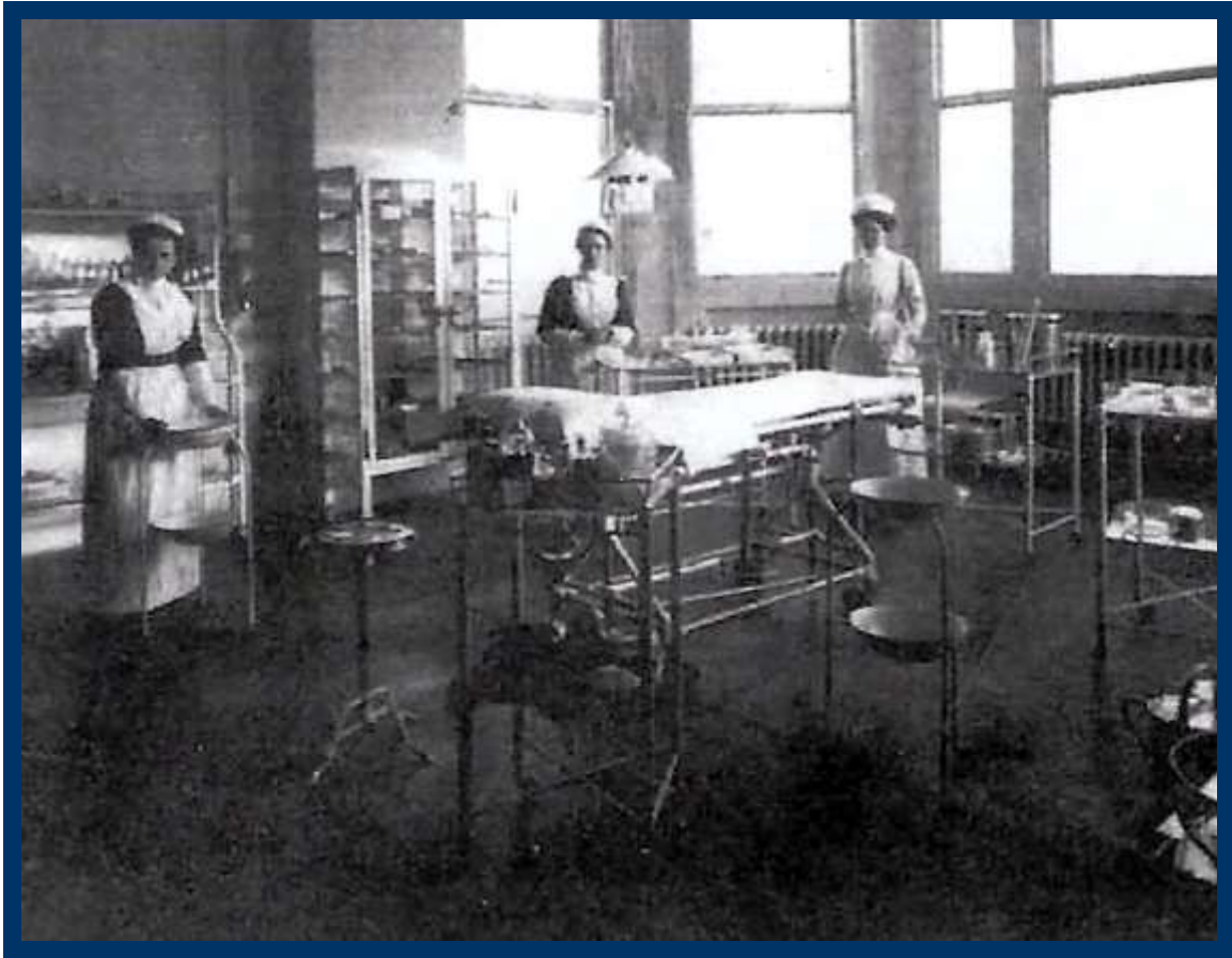
Opened in Winsor 1909, 50 beds, steel-framed building, heating by under-window radiators.
