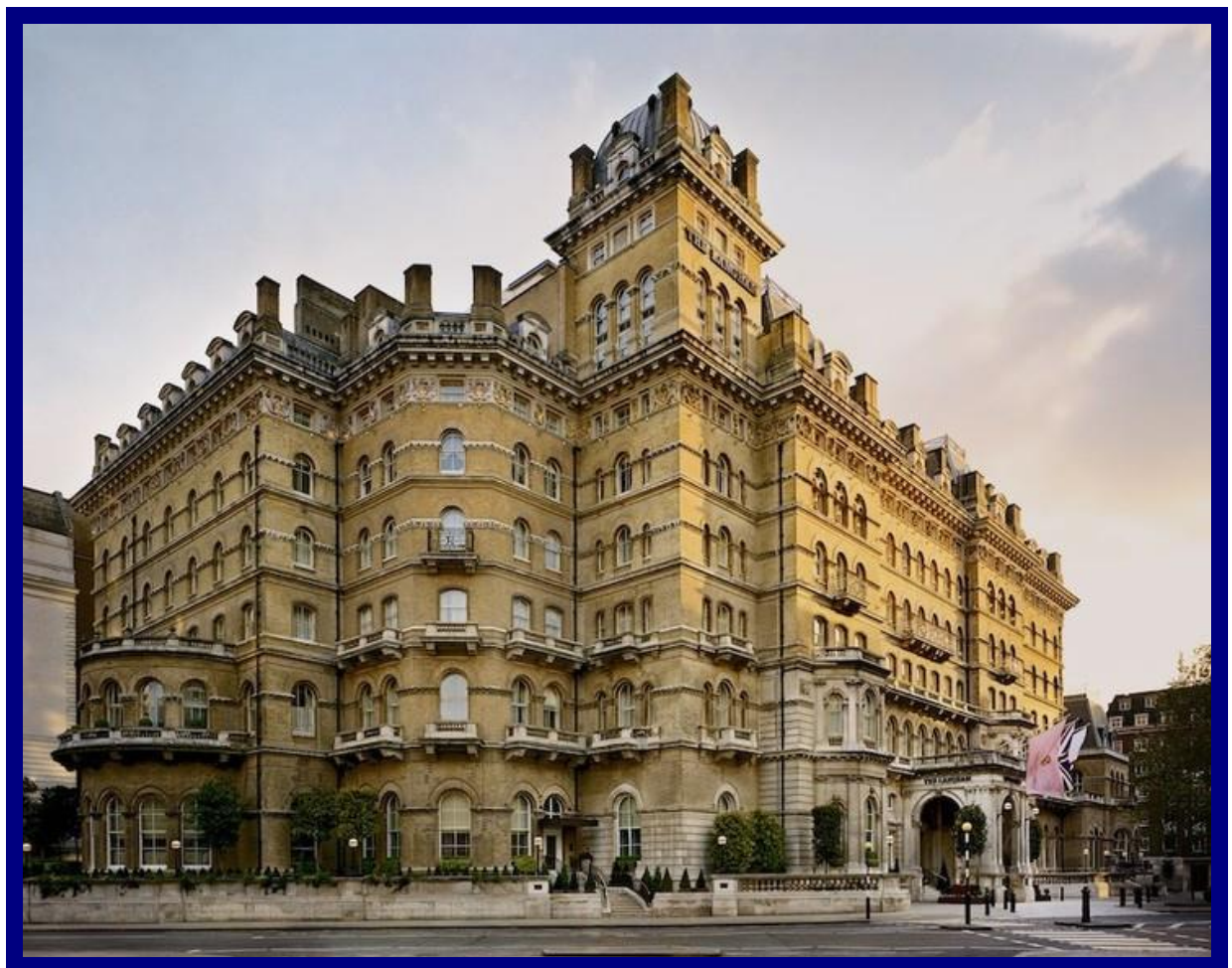
The Langham Hotel of 1865, with 100 water-closets and 36 bathrooms. Said to have England's first hydraulic passenger lift.
