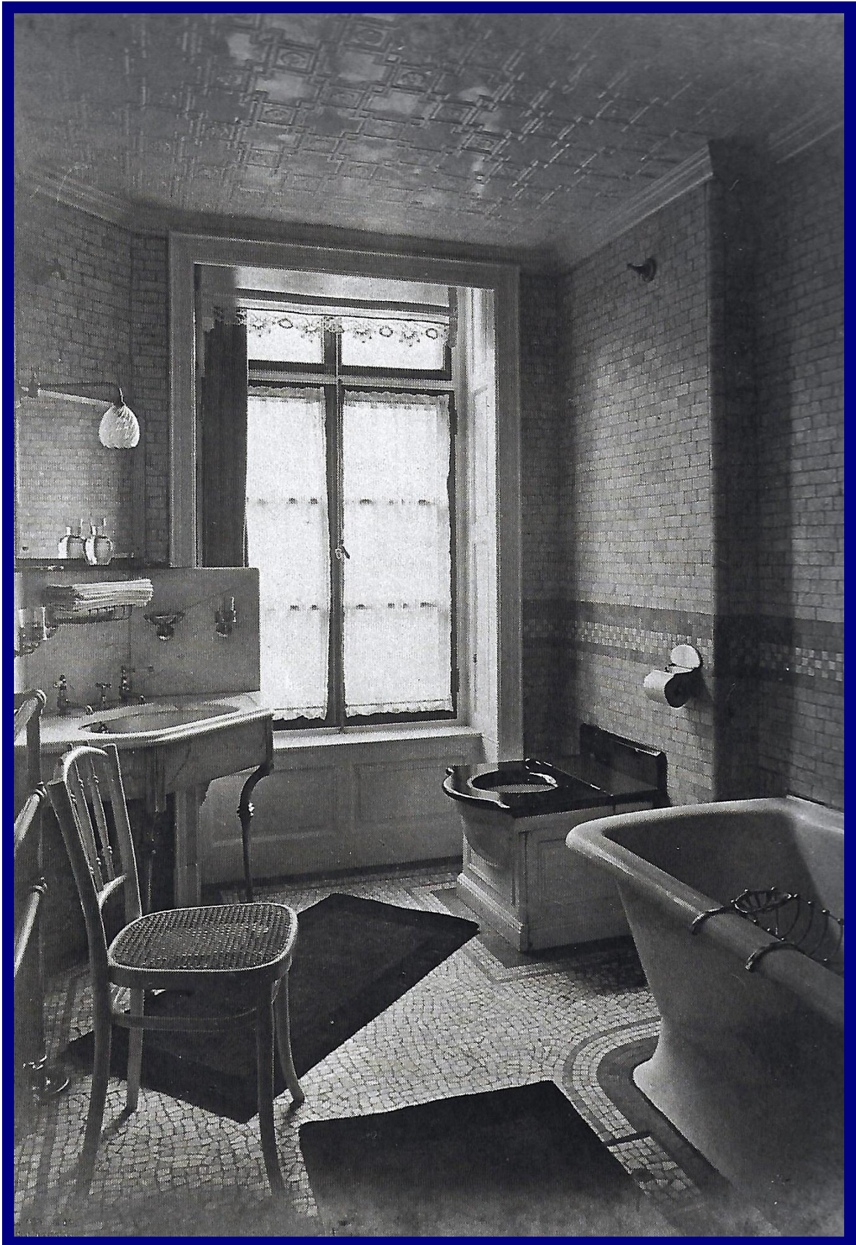
Savoy Hotel, London, built 1889, enlarged 1904. Heated corridors, 70 bathrooms. "Electric light everywhere and at all times. No gas. Large and luxurious lifts".
