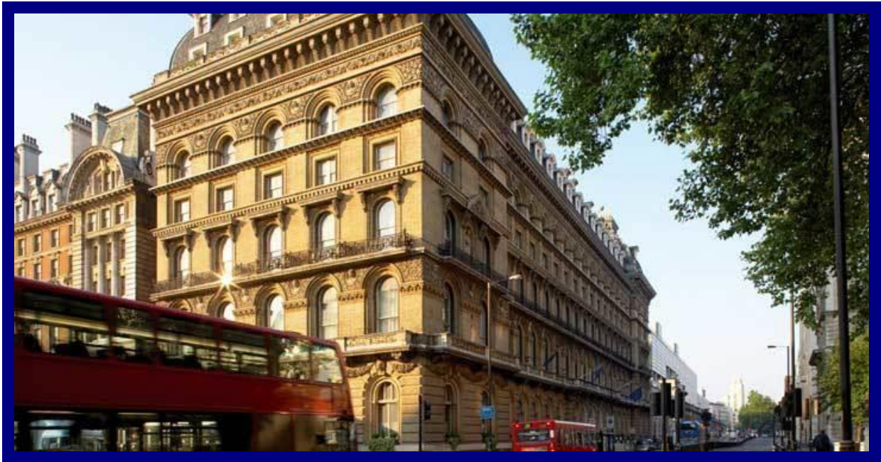
Grosvenor Hotel, opened in 1929. First London Hotel to have a bathroom for every bedroom. Once famous for its Great Room, originally an ice-rink.
