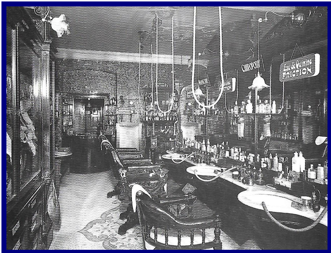
Barbers Saloon at the Hotel Cecil in London, 1911 (note the plumbing).
