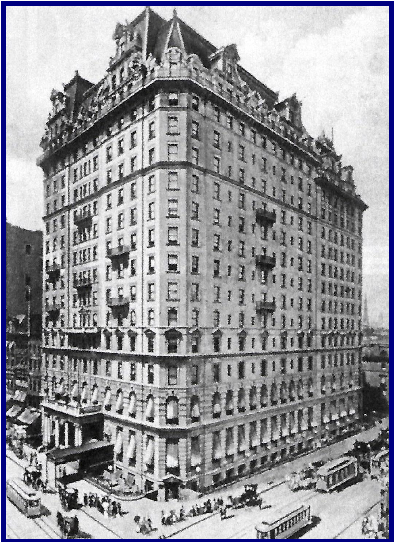
1896: 250 ft, 14 floors, for short time said to have been tallest hotel in world, demolished 1961.
