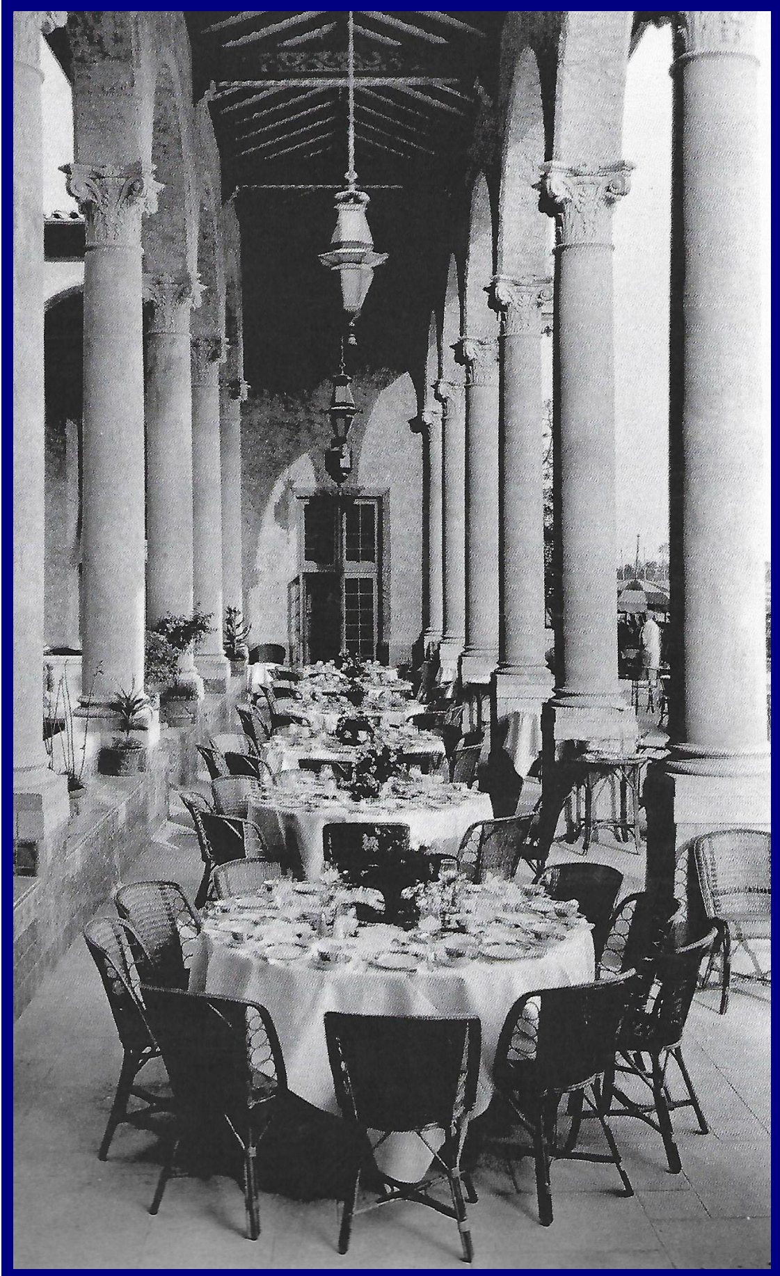
Terrace over the patio, c.1926.
