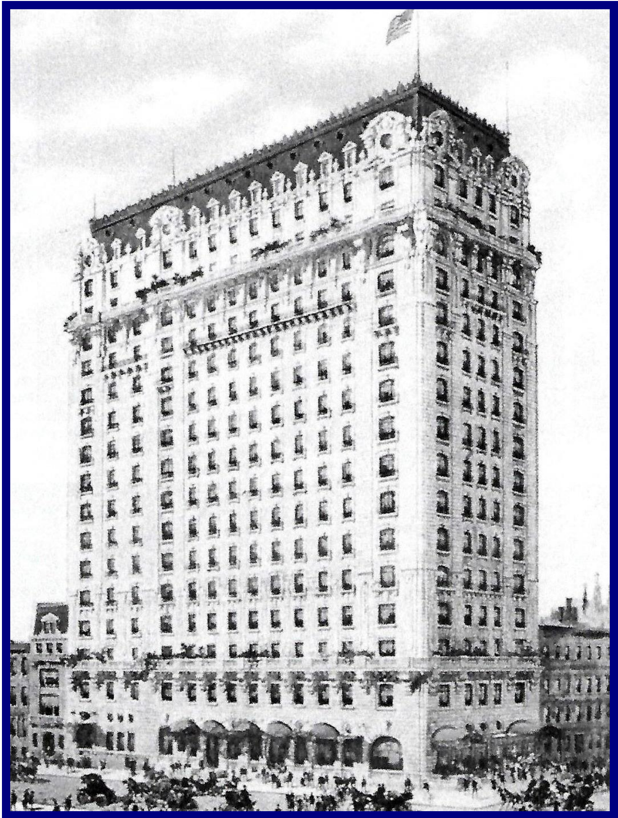
1904: 20 floors, 181 rooms & numerous condominiums, then New York's tallest hotel. Central vacuum cleaning system, electric clocks and heating thermostatic control.
