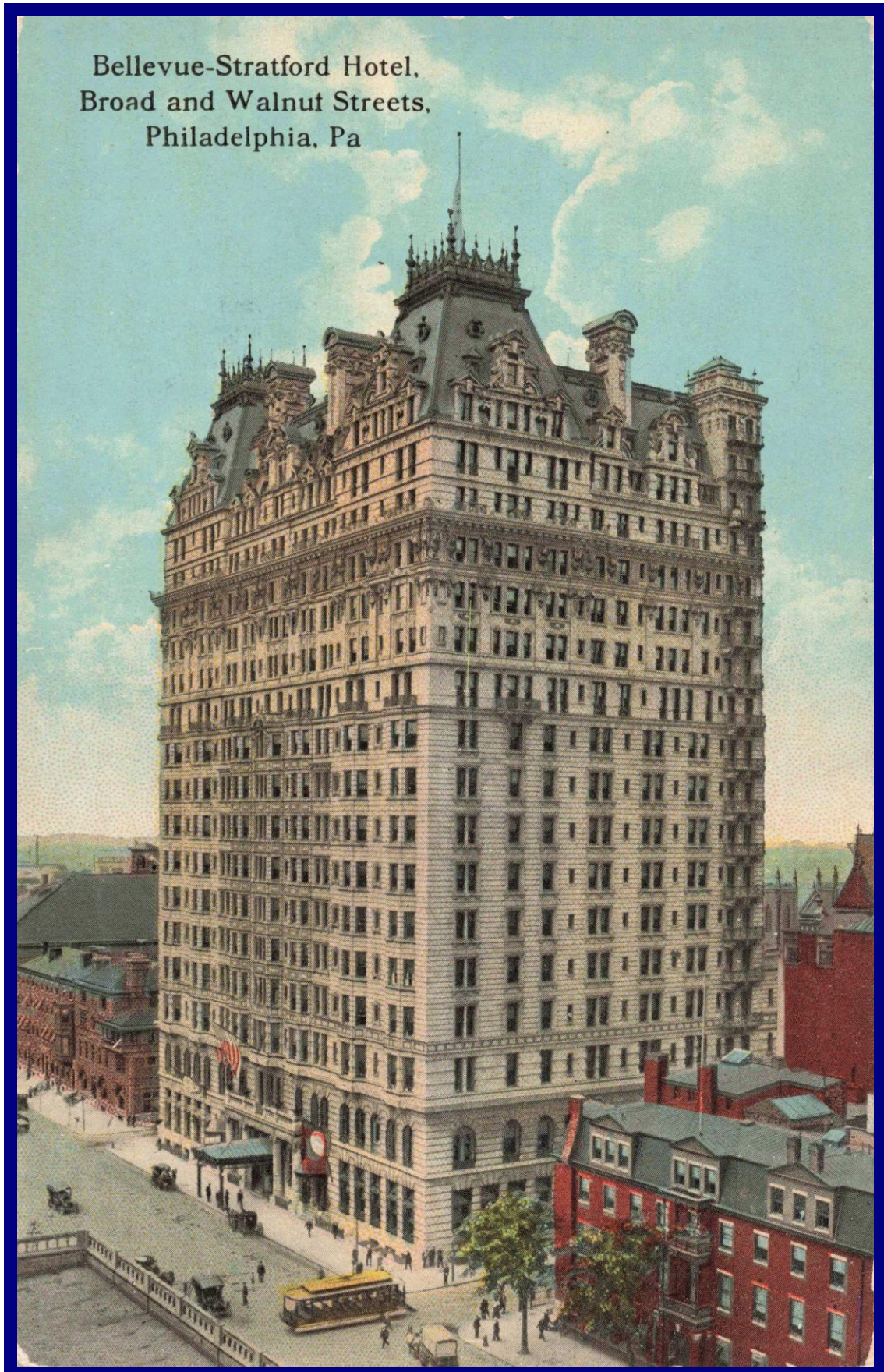
Built 1904, extended to 19 floors with 1090 rooms in 1912.
