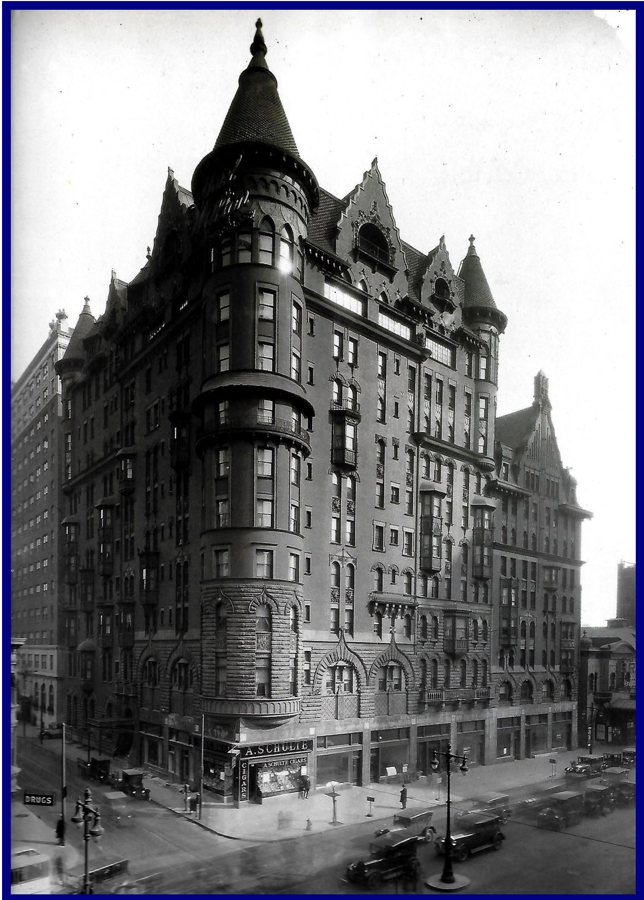
Built 1908, 11 floors, 146 ft, 400 rooms (200 baths). Architect: Angus Wade. Demolished 1966.
