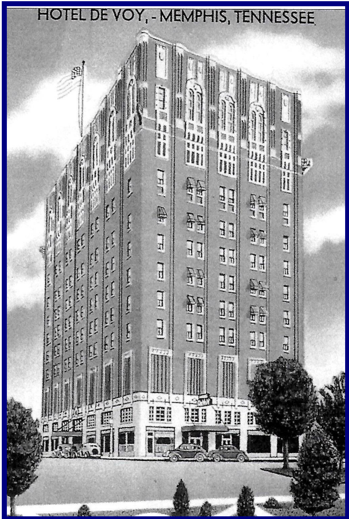
Originally Hotel King Cotton. Closed 1972, demolished 1984.
