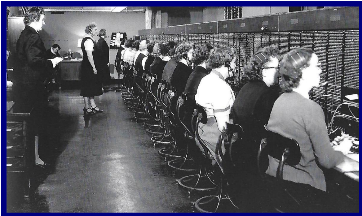
The hotel telephone switchboards in late 1950s with 17 operators handling 6 million calls a year.
