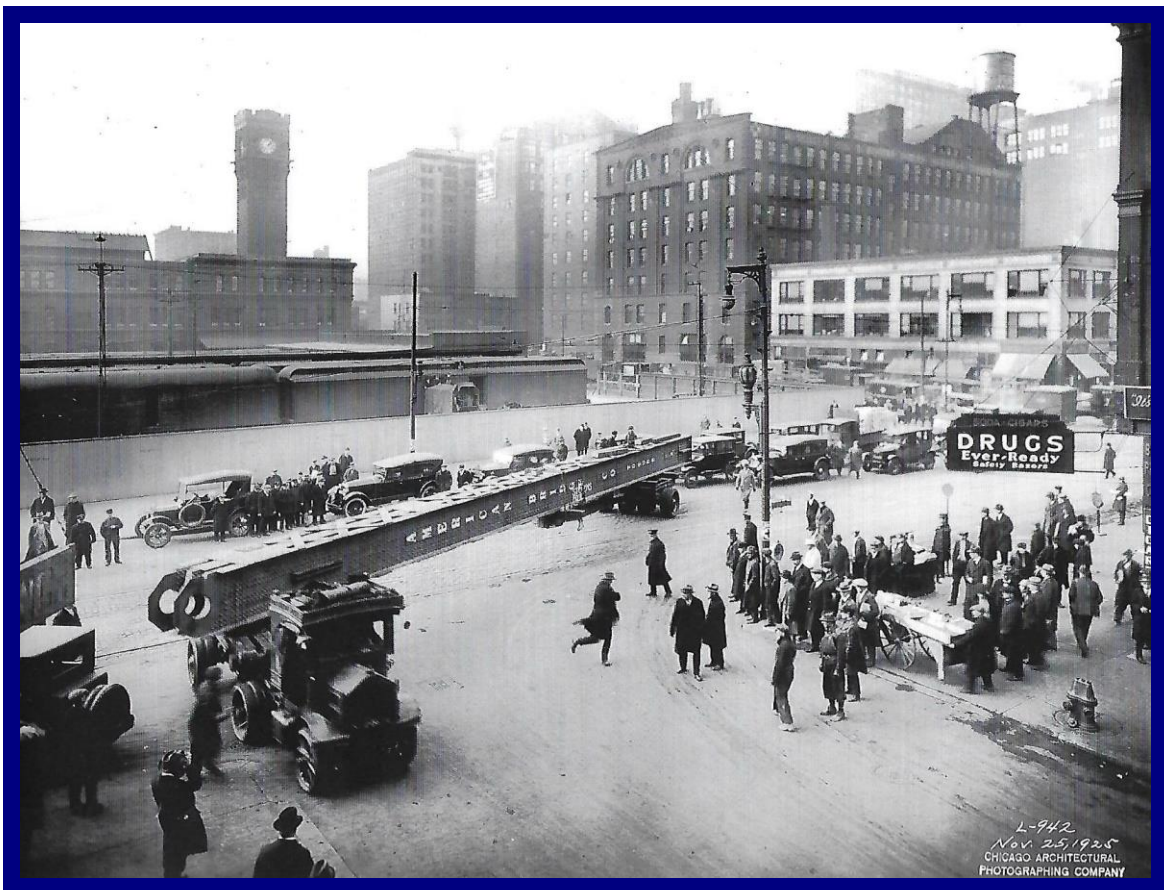
Under construction in 1925. The column being transported 77 ft long, weighing about 80 tons.
