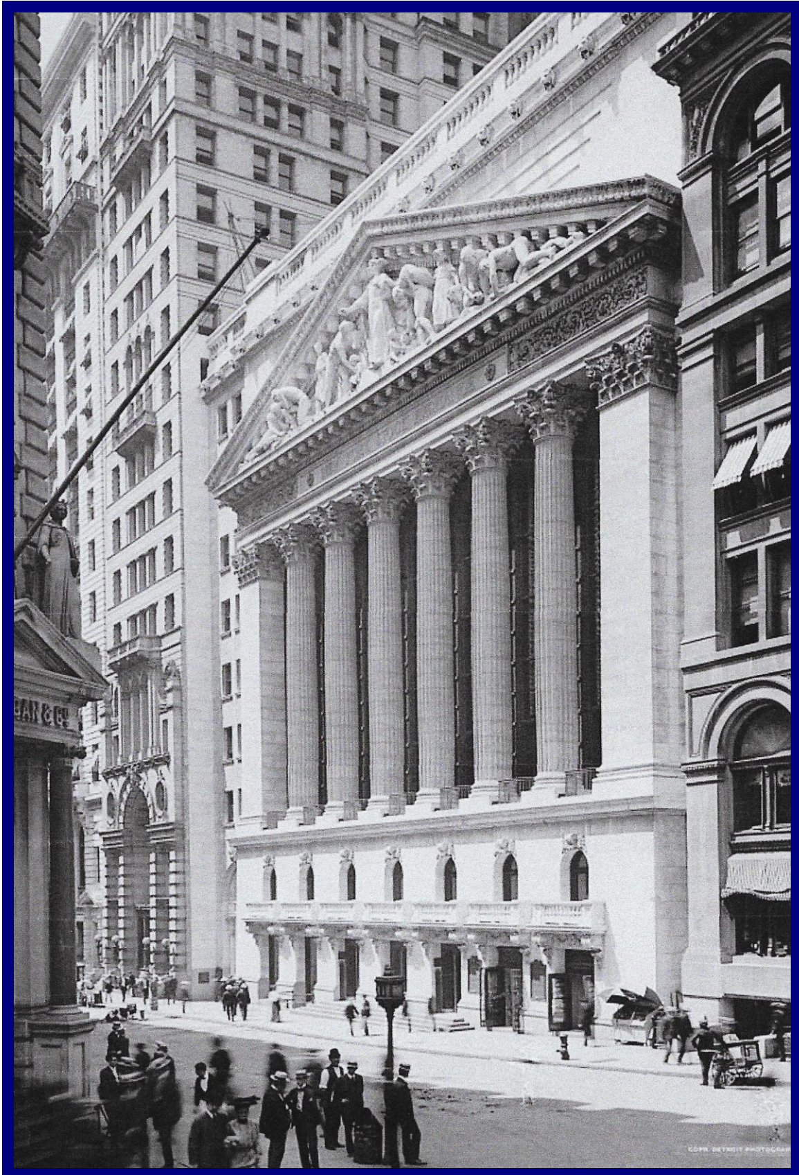
Photograph of 1904 from the Library of Congress. All fourteen storeys were mechanically ventilated (200,000 cu.ft/min). A detailed description is available in Arnold, pp.14-18.
