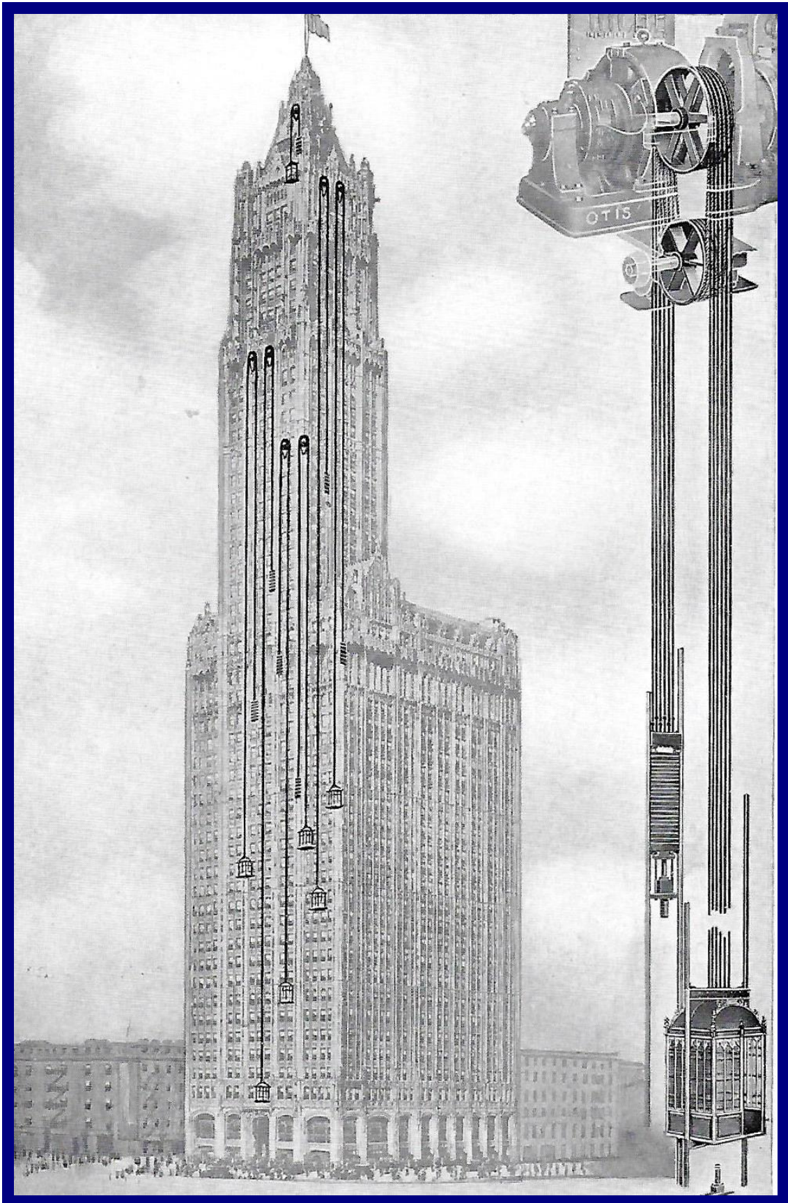
Provided with 29 Otis Electric Elevators. Six Tower elevators maximum capacity 3000 lbs, speed 700 ft/min at 2500 lbs. A seventh elevator runs from 53rd floor to Observation Station. Technical details of elevators and controls are in "Master Builders," pp.45-50.
