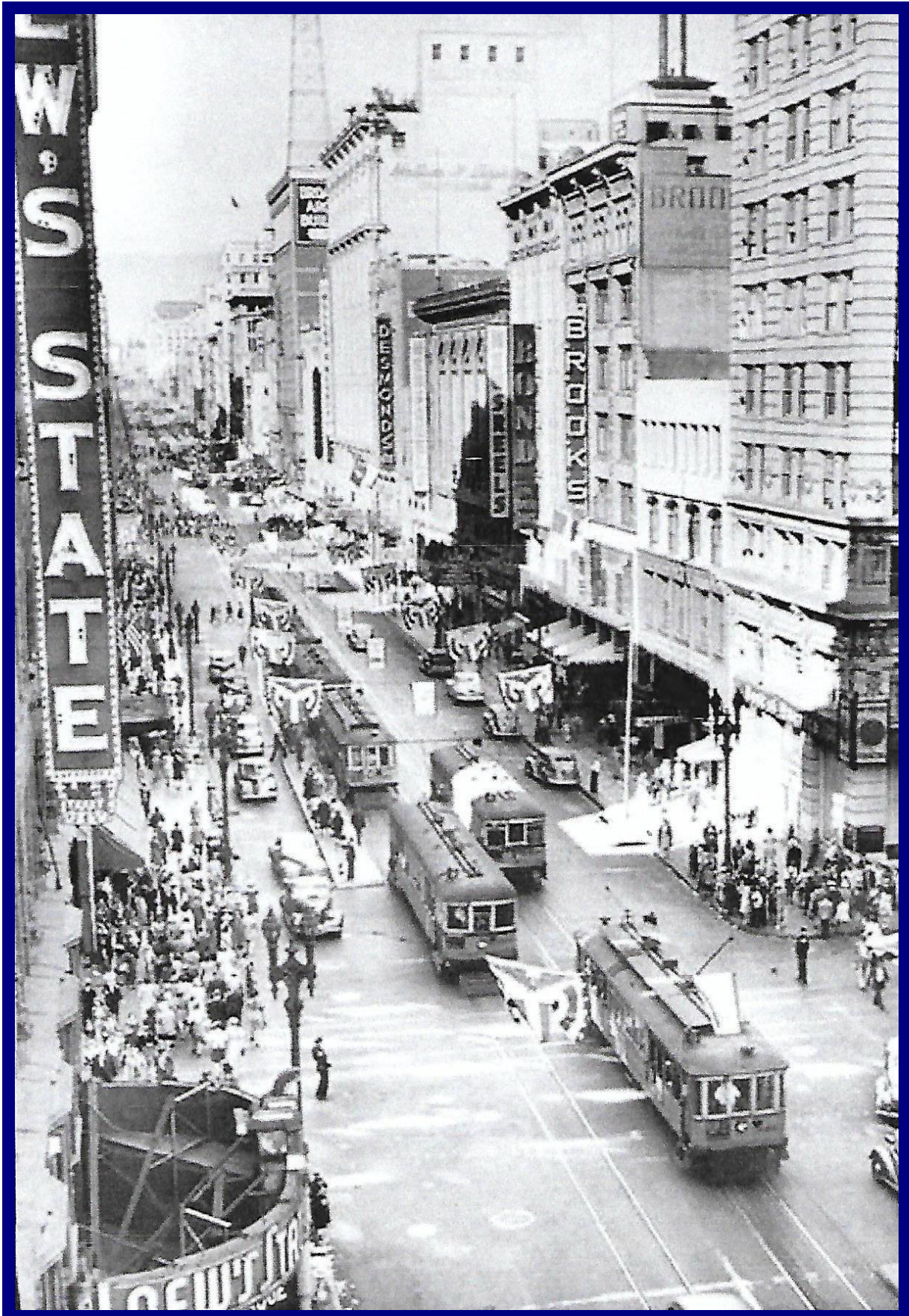
2422 seats. Air conditioned by the Wittenmeier Machine Company of Chicago, with CO2 refrigeration plant.
