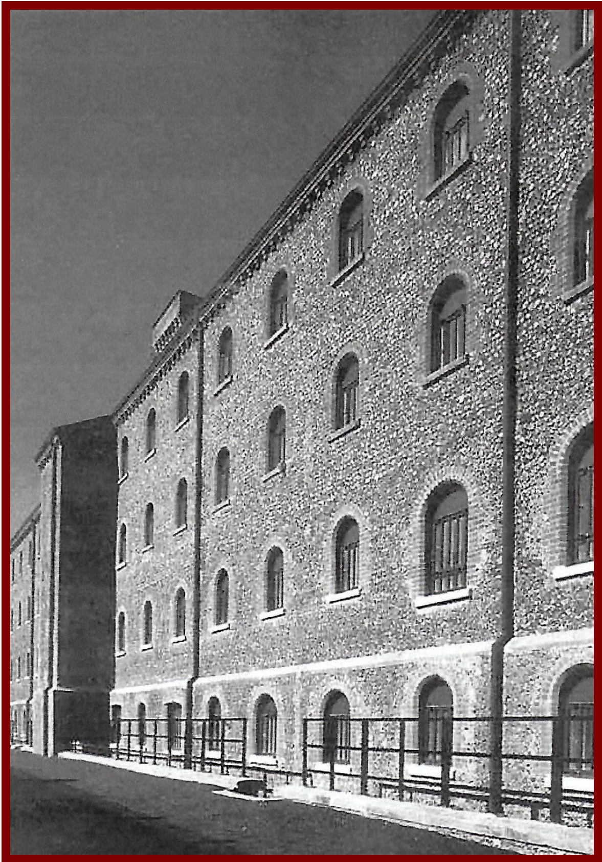
View of A-Wing, built 1852-53, D.R. Hill.
