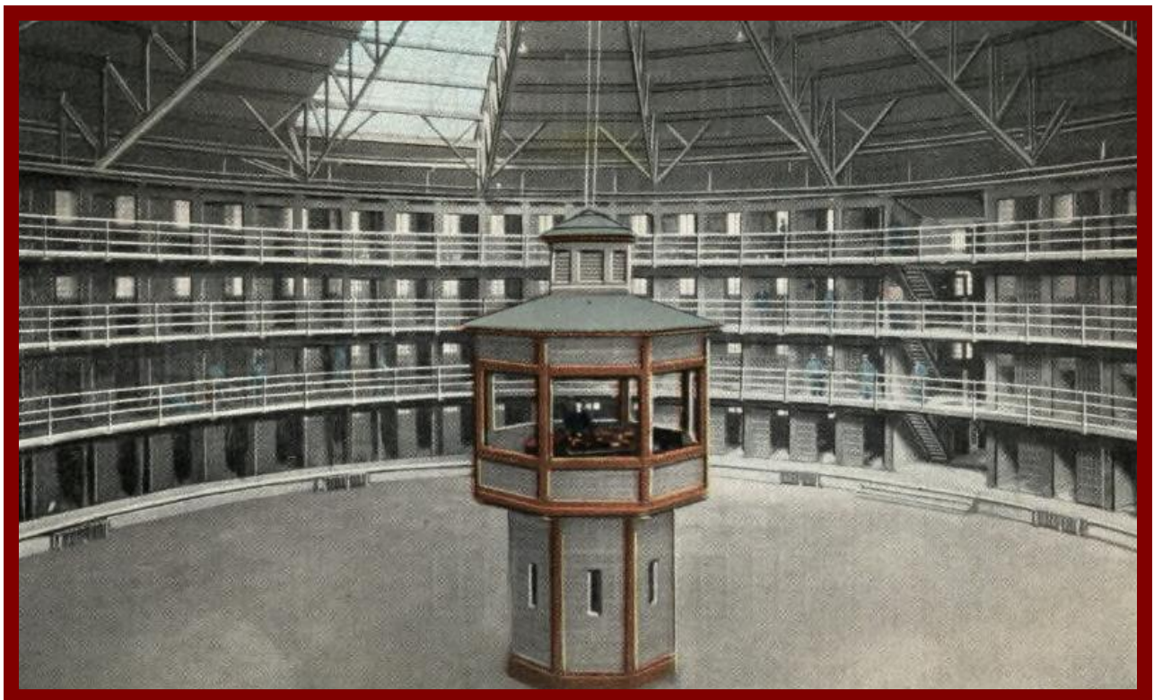
Central guard tower in open internal space surrounded by tiers of cells.
