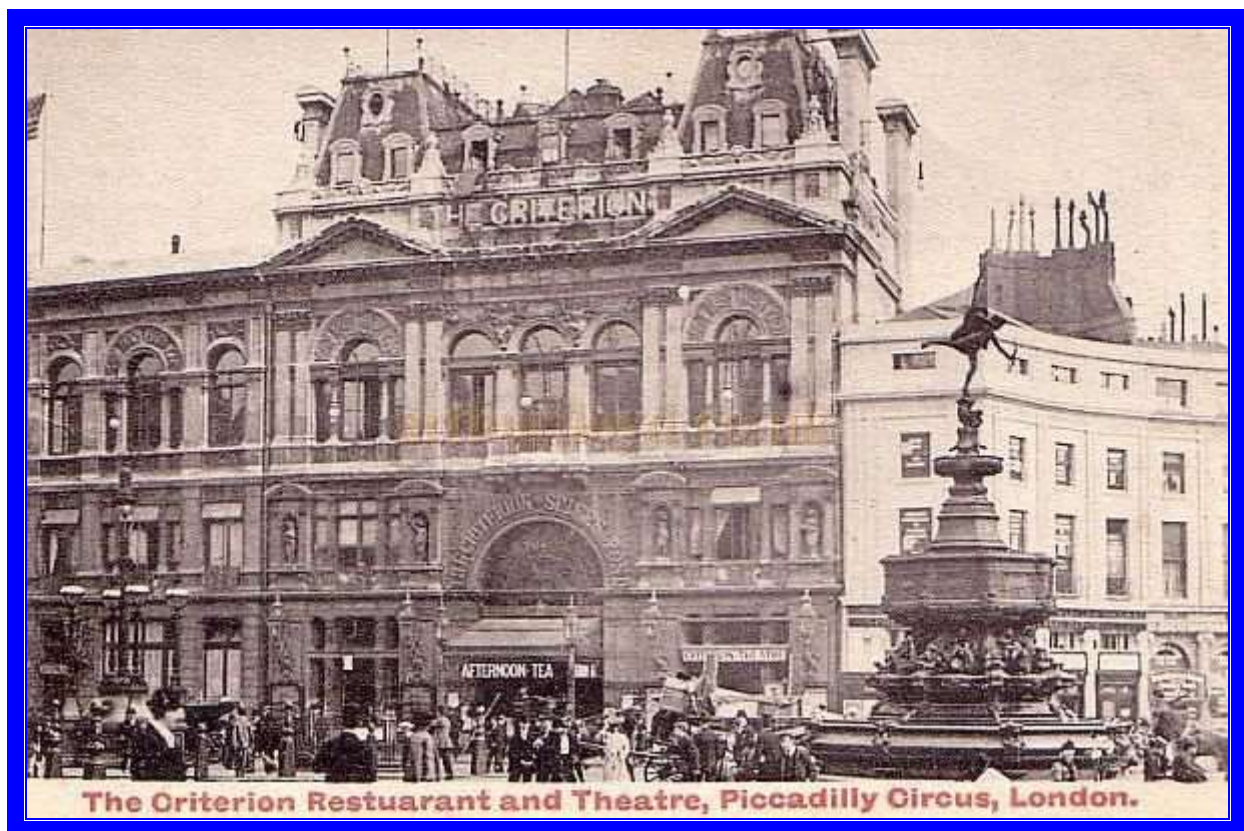
Criterion Theatre, London, 1872, reconstructed 1883 and 1903.
