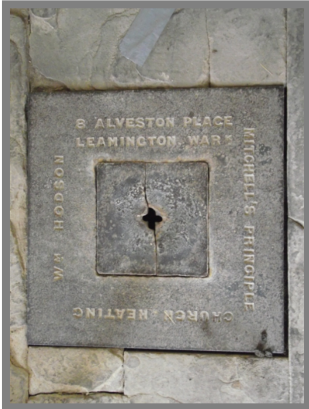
Cast iron floorplate with inscription and removable centre section
