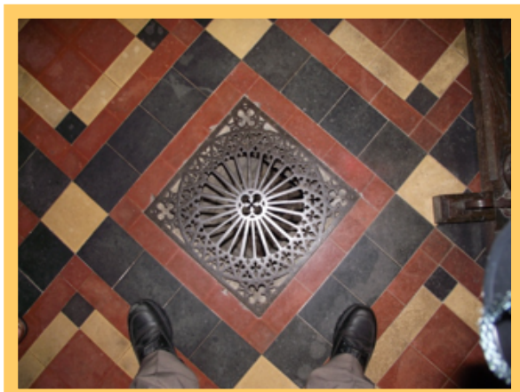
Cast iron floor grating for the warm air heating system
