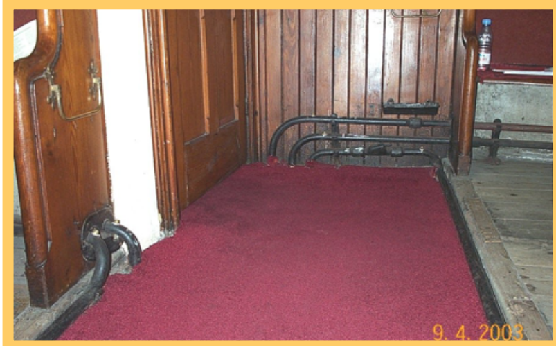
View at floor level of expansion loop in pipework
