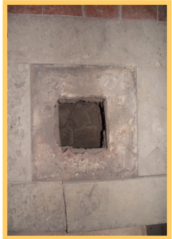
Floor plate removed looking into brickwork hot-fire pit
