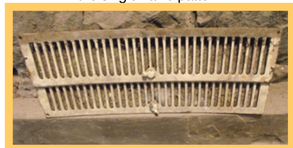
The Ventilator Grille shown above is the double valve pattern
