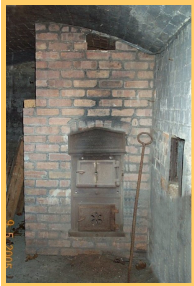
The warm air stove front plate in its original position with a cleaning tool
