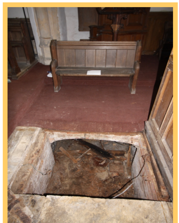
View into floor-pit facing the rear vaulted coal storage area.
