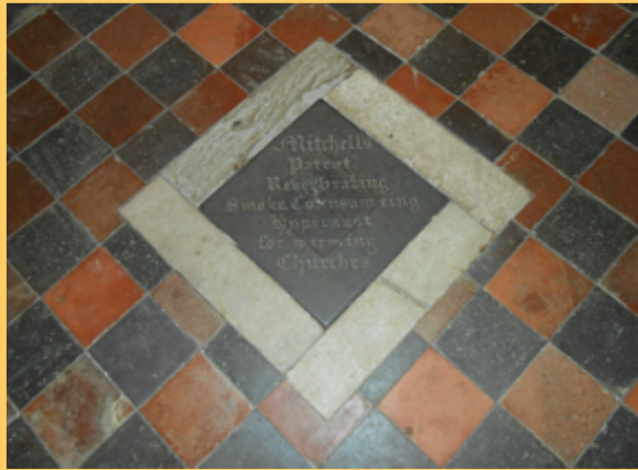
The wording on the remaining floor cover plate Mitchell's Patent Reverberating Smoke Consuming Hypocaust for Warming Churches
