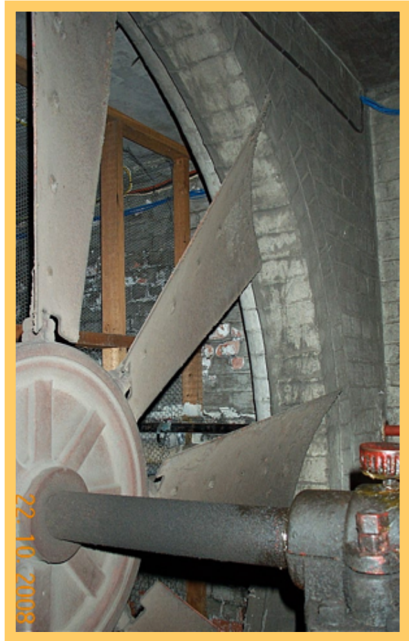
Note the curvature of the brickwork surround
