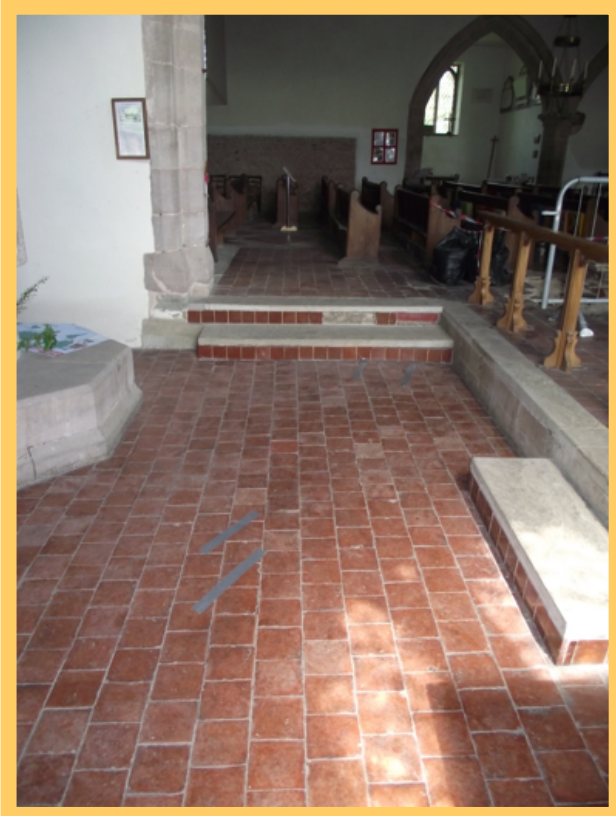
View across South Aisle showing marker tapes over floor ducts
