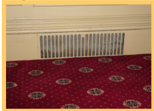
The ventilator grille shown above is the single valve pattern
