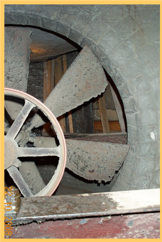
Belt drive with propeller fan blades
