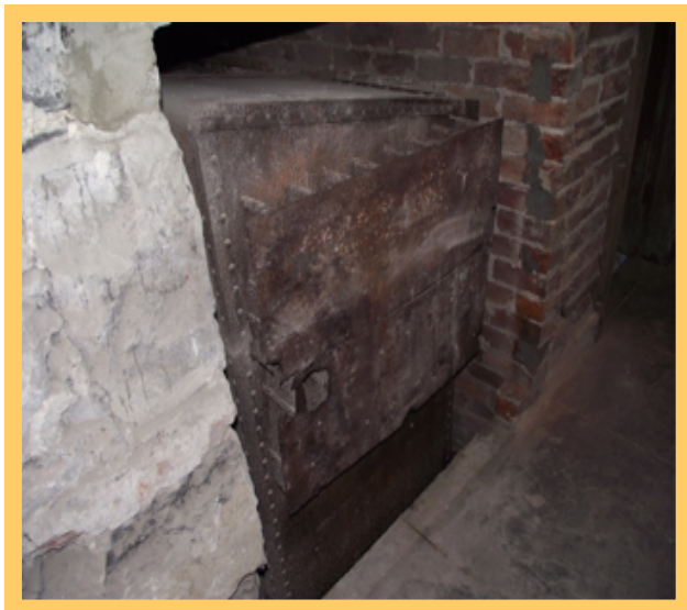
View looking from adjacent corridor after the wall had been removed
