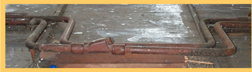
View at floor level of expansion loop in pipework
