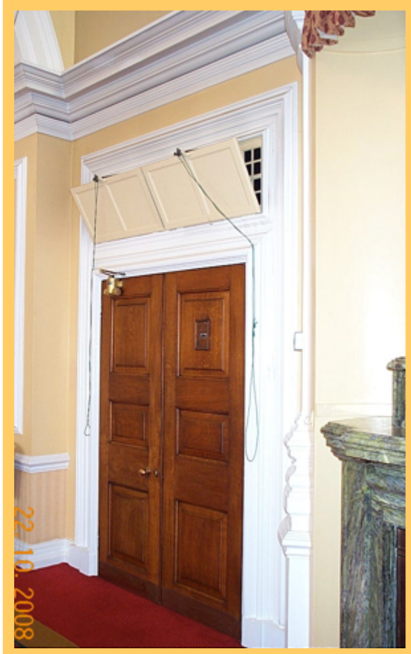
High level supply air inlet with flap dampers and pull cords
