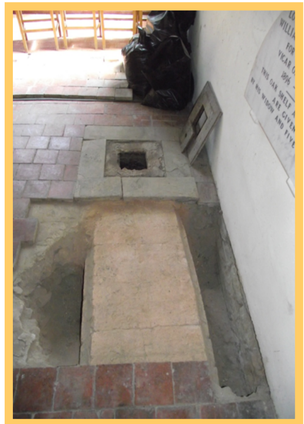
Section of the underfloor flue duct enclosed in brickwork
