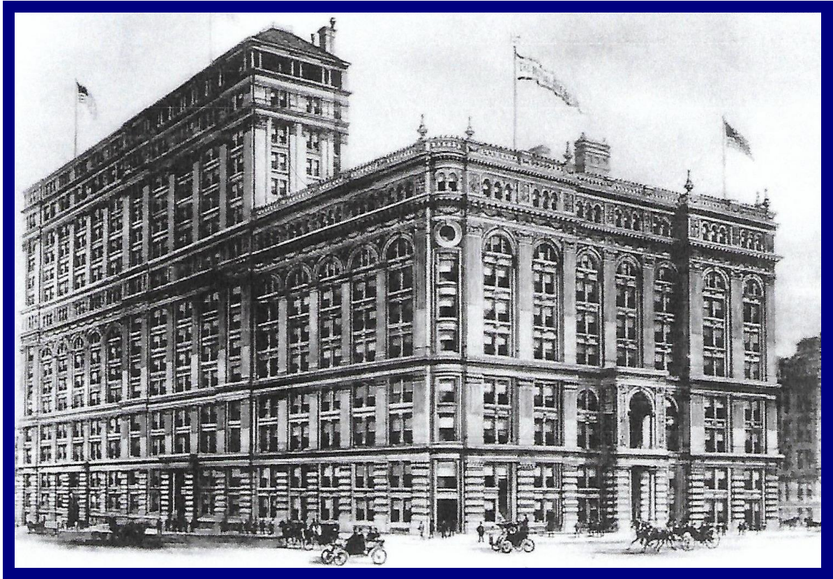
Mutual Life Insurance 1884. Under-window radiators with fresh air inlet ventilation and mechanical exhaust.
