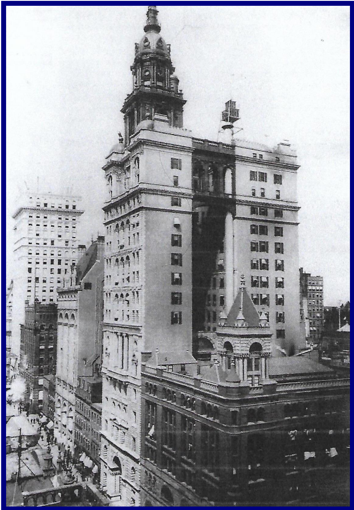
Under-window radiators, sash inlet ventilators and mechanical exhaust 1894. Note external window blinds.
