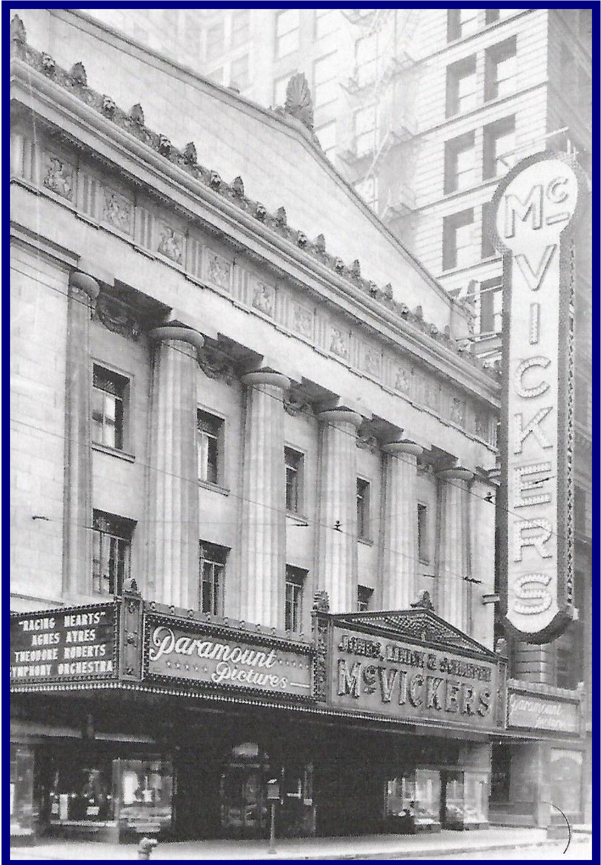
Air conditioned in 1924, designed by Otto Armspach, with Kroeschell CO 2 refrigeration.
