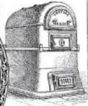
COTTAGE BOILER 50 FEET WATER RADIATION SUPPLIED 150 TO 200.
