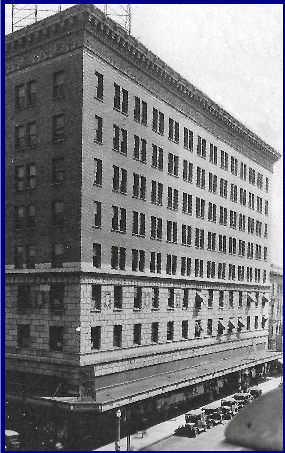
Existing building, air conditioned 1926, refrigeration Carrier centrifugal.
