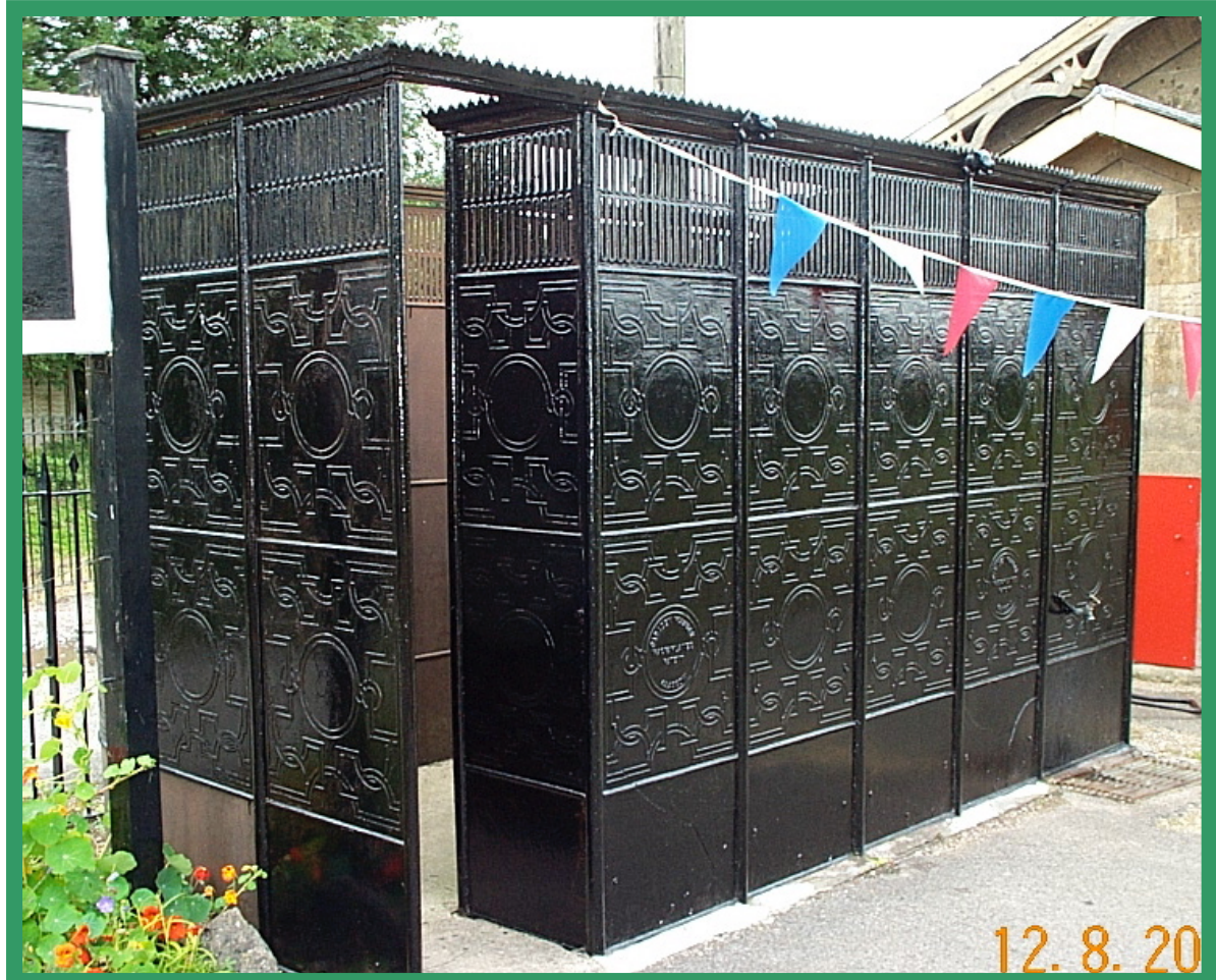
A fine example of a single doorway Urinal at the Cranmore Station of the East Somerset Preserved Heritage Railway in Somerset. The name of the manufacturer displayed on one front panel is Walter Macfarlane of Glasgow made at their Saracen foundry
