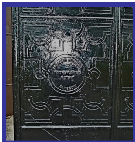
A fine example of a single doorway Urinal at the Cranmore Station of the East Somerset Preserved Heritage Railway in Somerset. The name of the manufacturer displayed on one front panel is Walter Macfarlane of Glasgow made at their Saracen foundry
