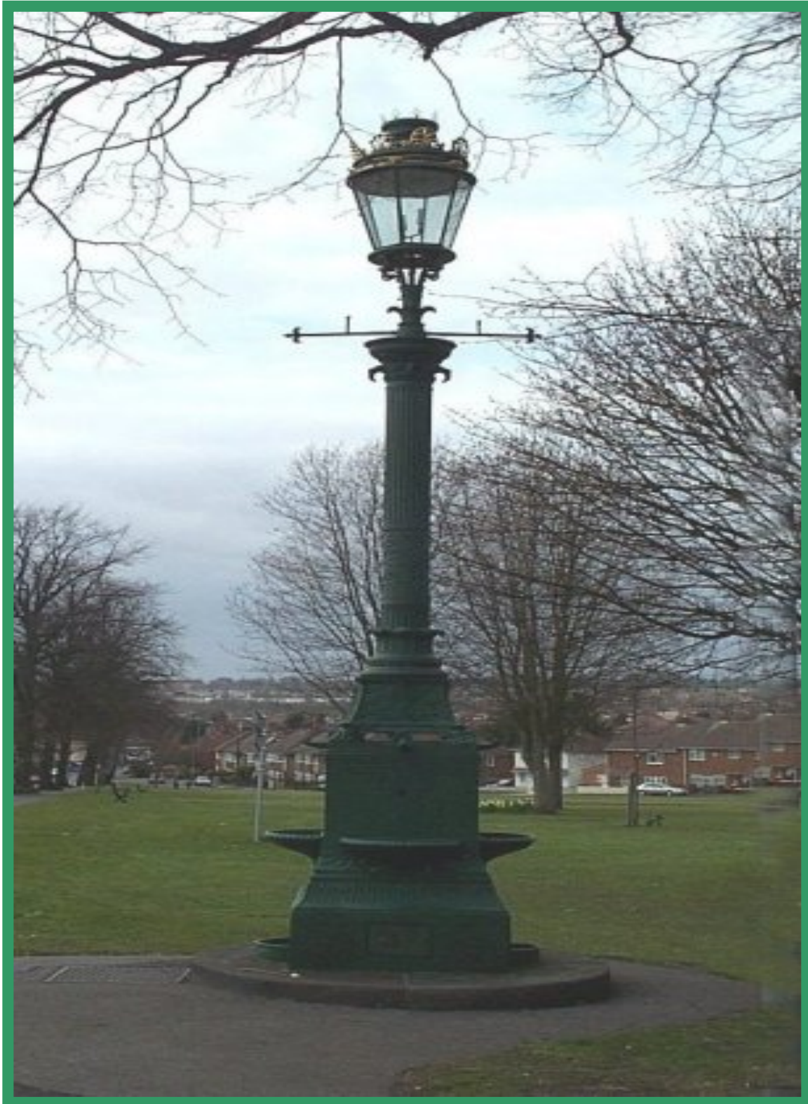
This cast-iron pedestal drinking fountain with light lantern was erected in 1900 and is to be found on a corner of Horfield Common in Bristol.
