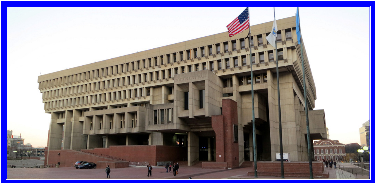
Opened in 1968, the Boston City Hall had an early Variable Air Volume air conditioning system
