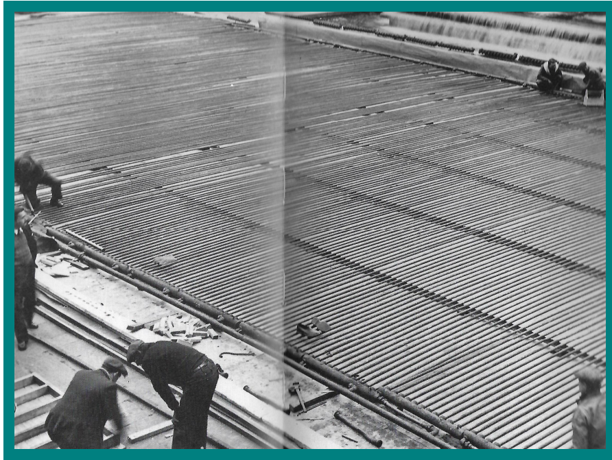
Laying the ice-rink piping grid (from "Works in Progress")
