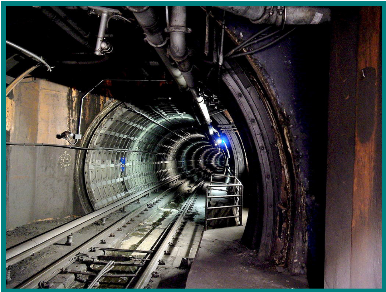
Typical BART tunnel section
