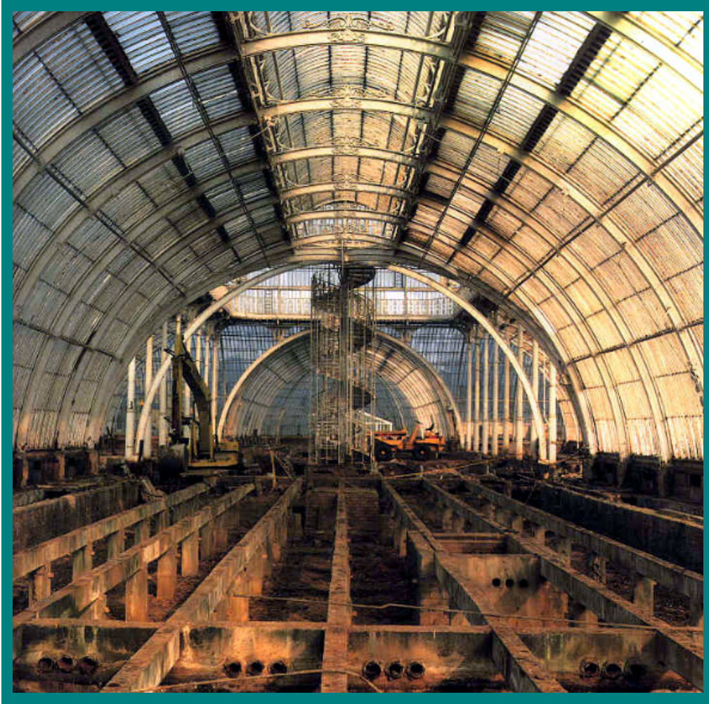
Restoration underway in October 1985, the underfloor heating pipes having been removed
