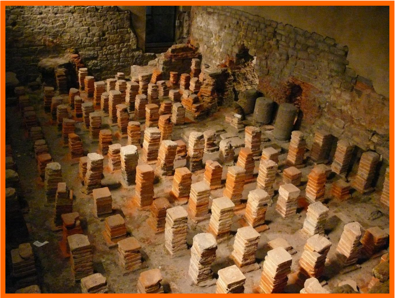
The tile pillars of the Bath hypocaust which once supported the floor above.
