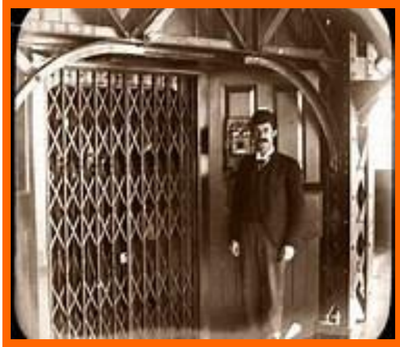
An original Tower hydraulic passenger lift.
