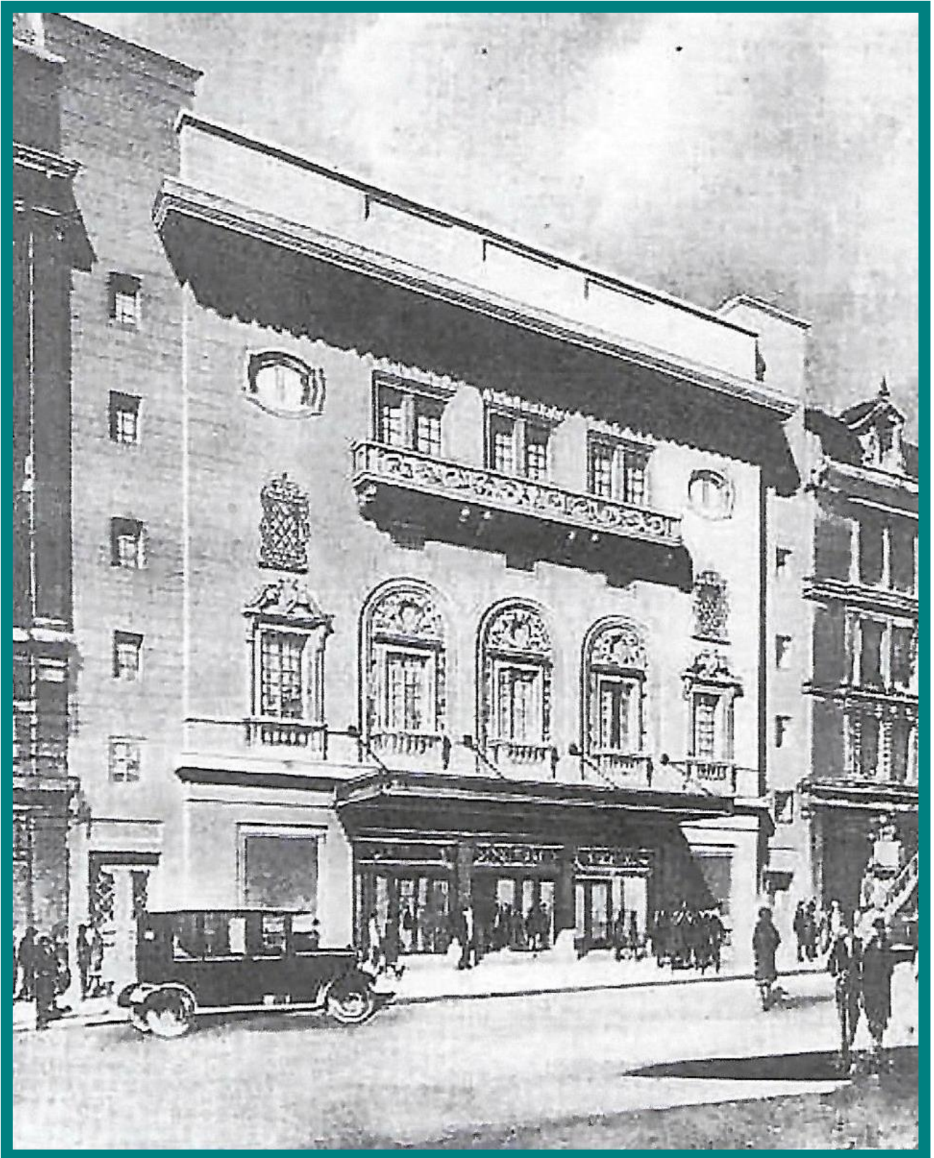
The Carlton Theatre (1159 seats) in the Haymarket in London, opened in 1927. Said to be the first fully air-conditioned theatre (i.e., with refrigeration) in Britain and with only the country's 4th Carrier centrifugal installation.
