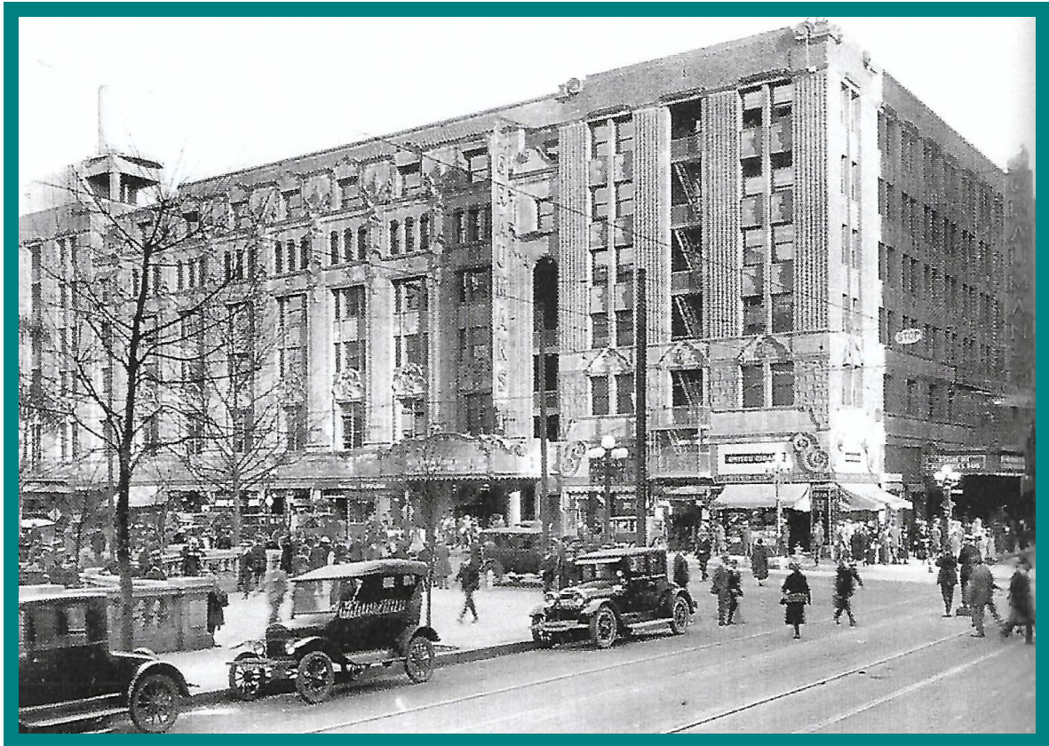
Metropolitan Theatre (3485 seats) 1921-22, first Carrier "upside-down" air distribution.
