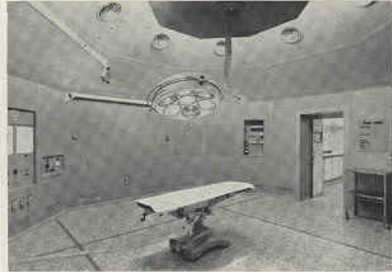
MODULAR OPERATING THEATRE AT HAMMERSMITH HOSPITAL FOR MEDICAL APPARATUS DIVISION OF HONEYWELL CONTROLS LTD.
