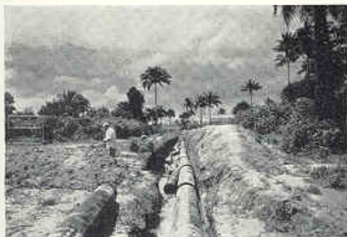
MICHELIN (NIGERIA) LTD., PORT HARCOURT, NIGERIA. Services provided by Brightside include air conditioning, ventilation, compressed air, process refrigeration plant, and all piping services throughout the factory. The refrigeration plant consists of two centrifugal machines with a total capacity of 880 tons of refrigeration. Condenser cooling water was piped through 2½ miles of jungle in 24 in and 16 in diameter tubing. Consultants: Michelin Tyre Co. Ltd., Stoke-on-Trent.
