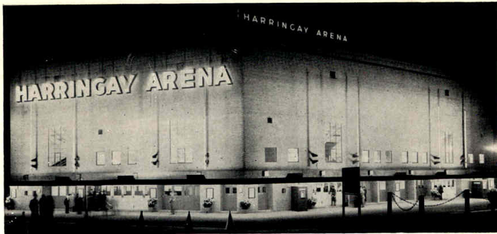
At Harringay Arena the installation was carried out by Drake & Gorham Ltd. Main switchgear was constructed at the Acton factory.
