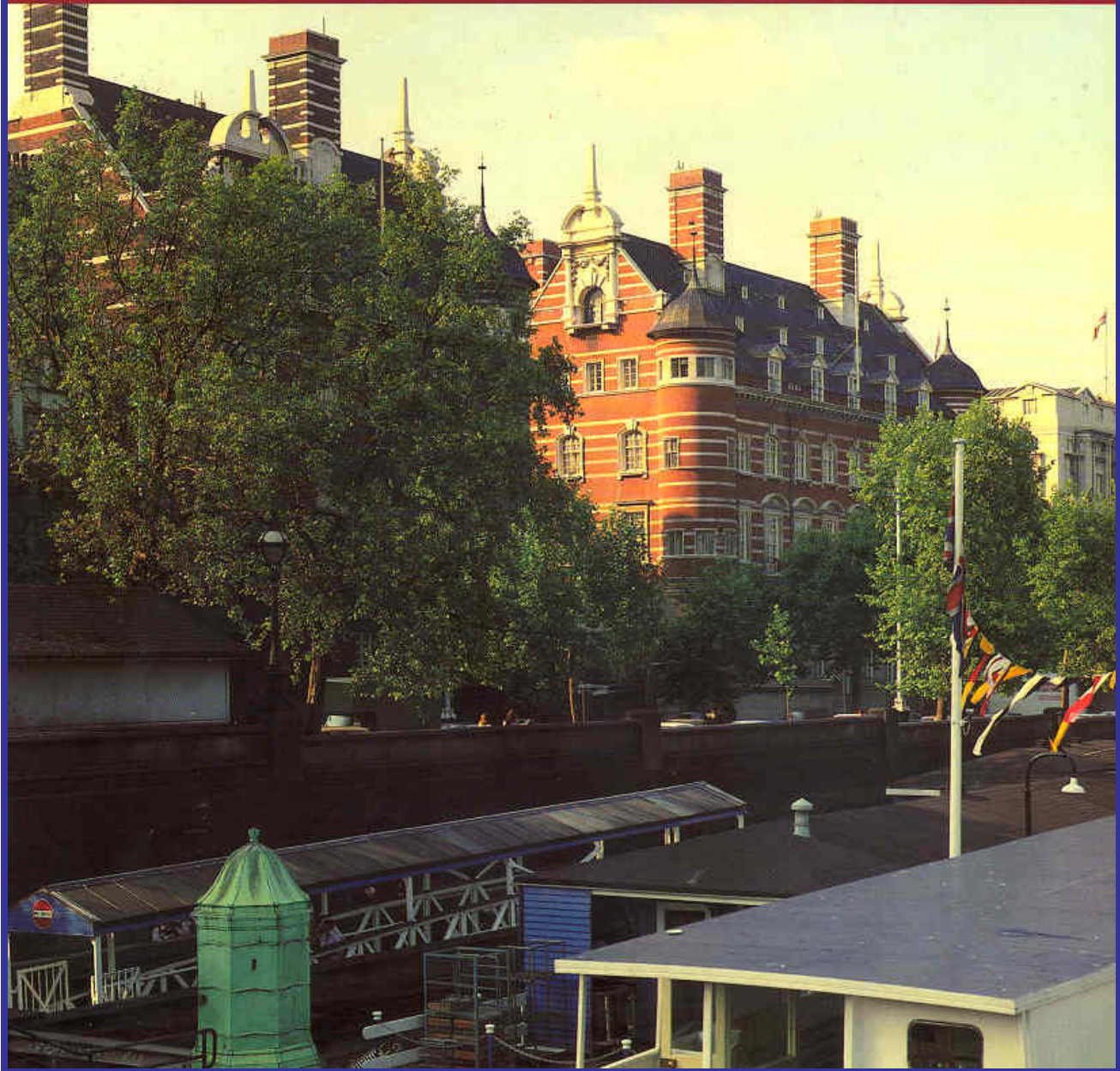
Norman Shaw Building (Old Scotland Yard), Embankment, London
