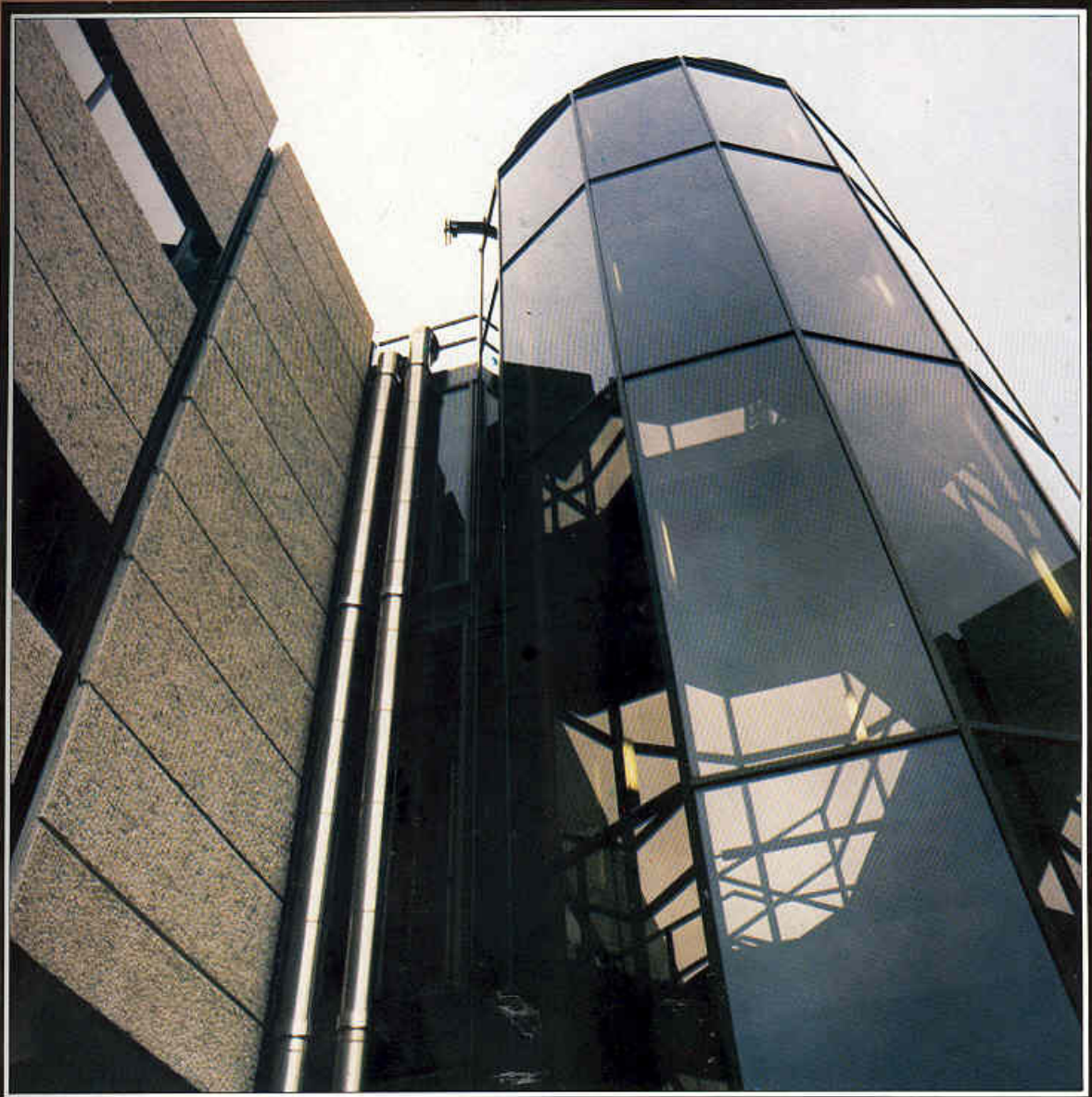
Above / IBM United Kingdom Limited, Havant / Drake & Scull was responsible for the installation of air conditioning, heating and plumbing services to Phases 6 and 7 of this manufacturing plant. Under the contract, the power house and satellite plant rooms were upgraded to accommodate the new facilities. Photo shows the chilled water pipework rising externally, adjacent to the west escape staircase.
