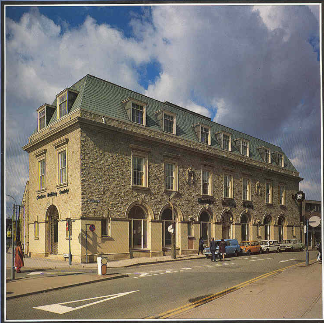
Top / Cheshire Building Society, Macclesfield / This contract comprised the installation of lighting, small power, fire alarm, communication systems, wiring to the VDU terminals and processors, air conditioning, plumbing and heating services.
