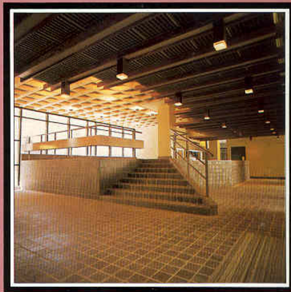
Above / Registrar General Building, Mauritius / Photos show a section of staircase and bar in the Banqueting Hall and part of the main plant room within the complex where Drake & Scull was awarded the design and installation of all mechanical, electrical, public, fire protection and air conditioning services.
