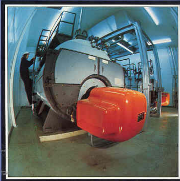
Top / Willis, Faber & Dumas Ltd., Head Office, Ipswich / The mechanical services for this project were installed by Drake & Scull, and included air conditioned office areas, with heating supplied by natural gas fire boilers and separate systems for the data processing computer and electronic telephone exchange.
