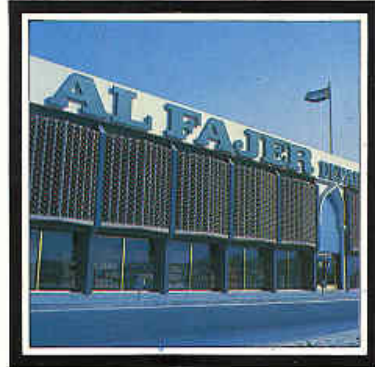
Above / Al Fajer Department Store, Dubai, U.A.E. / The electrical contract completed by Lunar Drake & Scull (U.A.E.) comprised the installation of general lighting, standby generator systems and fire protection systems for this 19 department, two-storey department store, one of the biggest of its kind in the U.A.E.
