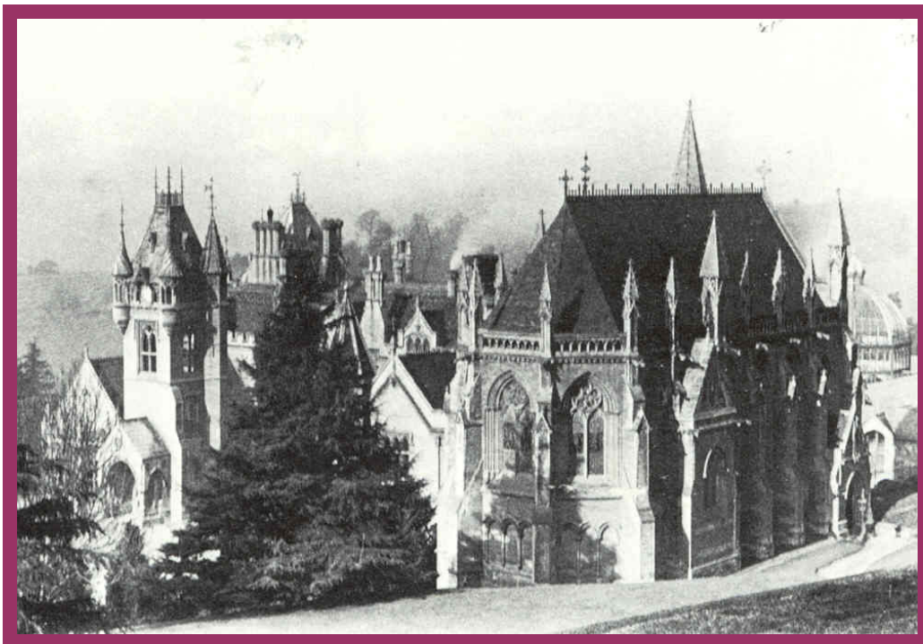
Built 1866 Tyntesfield, Wraxall, near Bristol G N Haden & Sons installed a hot water heating system, probably in the 1880s Architect John Norton
