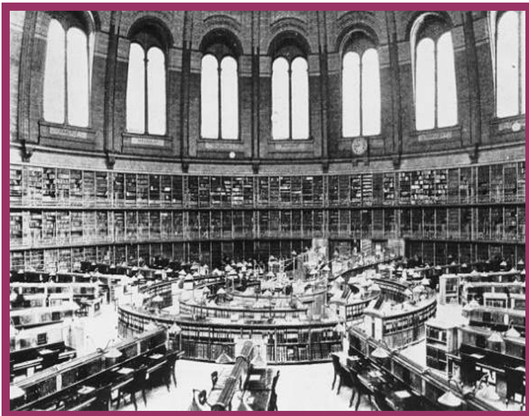
1858 British Museum Reading Room, London Hot water heating by G N Haden The architect was Sydney Smirke
