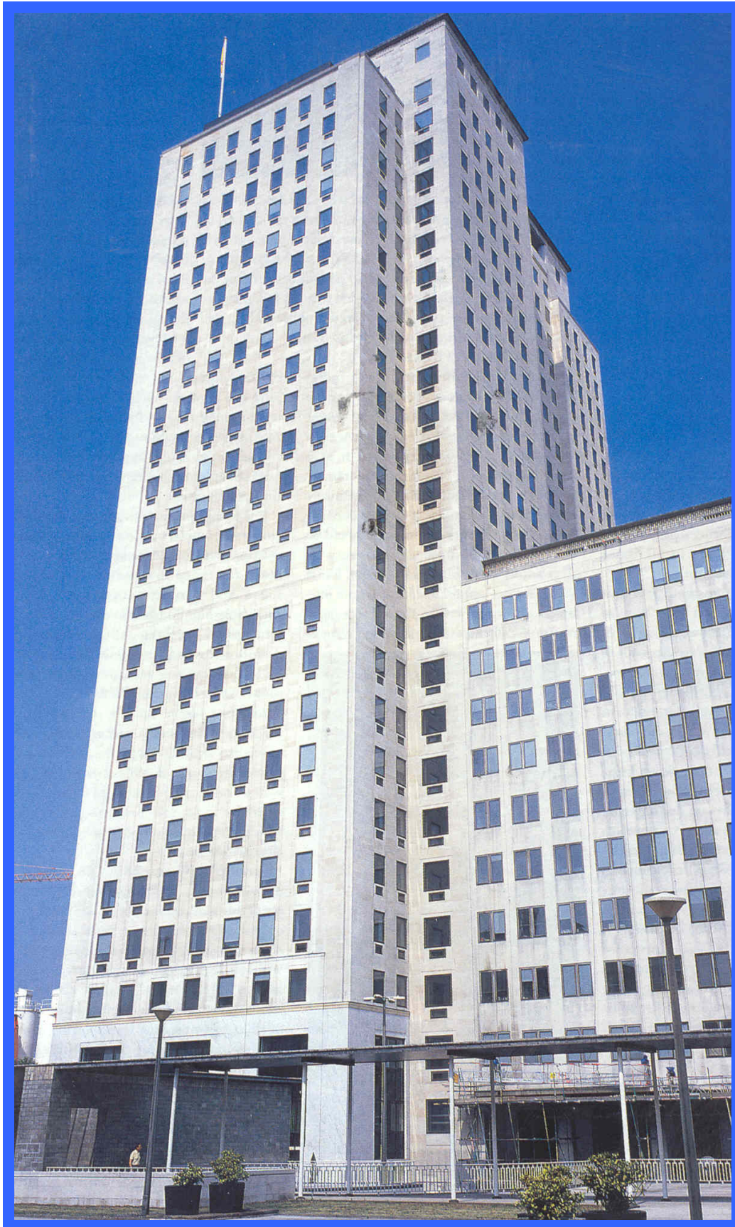
1962 Shell Centre, London. Then the largest air conditioned office block in Europe Chilled radiant panel ceilings (2700 TR refrigeration)
