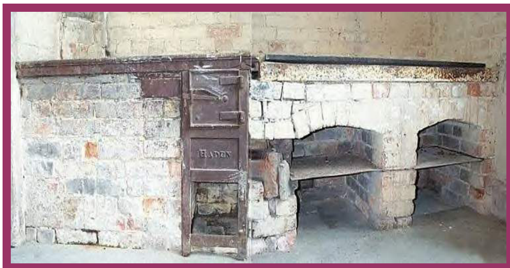
1830 G & J Haden installed heating stove and oven in Dinton House [Photos Frank Ferris]
