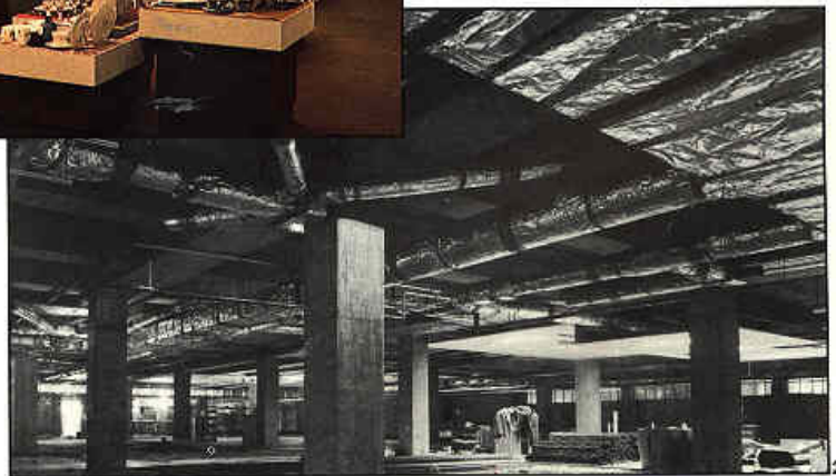
1 & 2 The finished ceiling conceals a labyrinth of services
