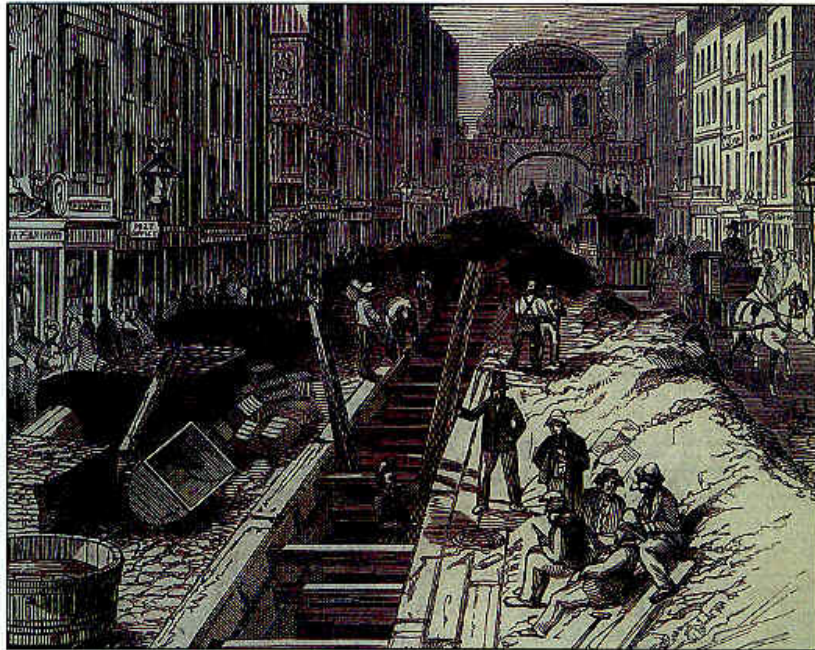
Deepening the sewer in Fleet Street, London, 1845
