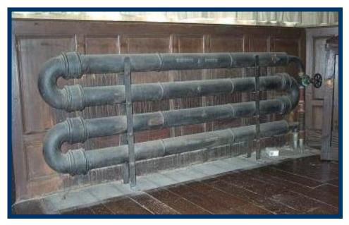
Cast iron pipework heating coil marked "W Sparrow, Martock" [Montacute House, near Yeovil, Somerset]
