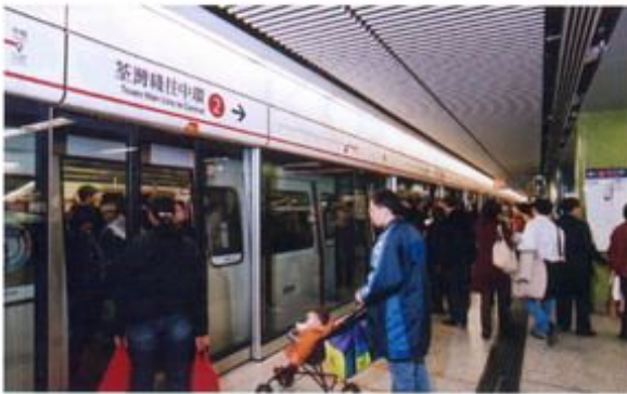
Jordan Station completed in 1979 and retrofitted with platform screen door in 2001
