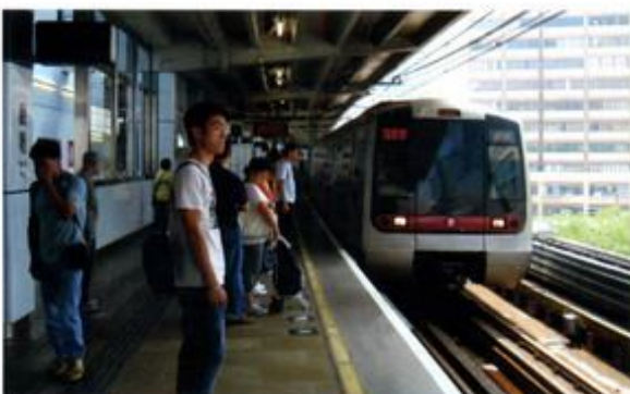
Kwun Tong Station completed in 1979, an above ground station utilizing natural ventilation for the platform
