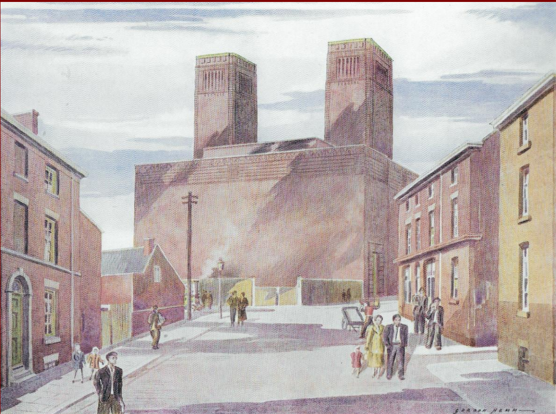
Sidney Street, Birkenhead, Ventilation Station
