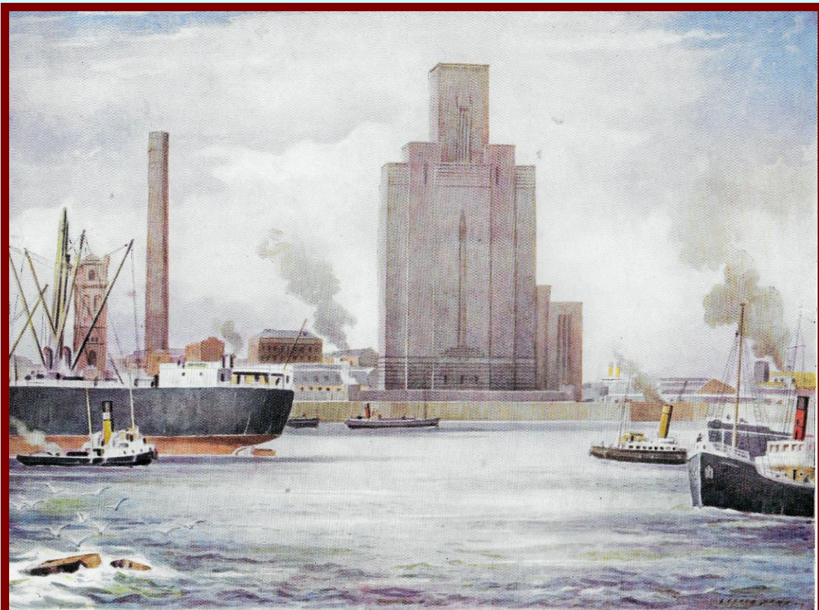
The Ventilation Station at Woodside, Birkenhead, as seen from the river
