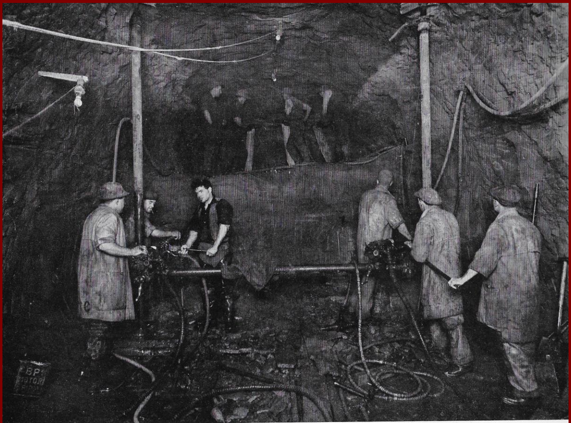
The driving of the pilot headings
