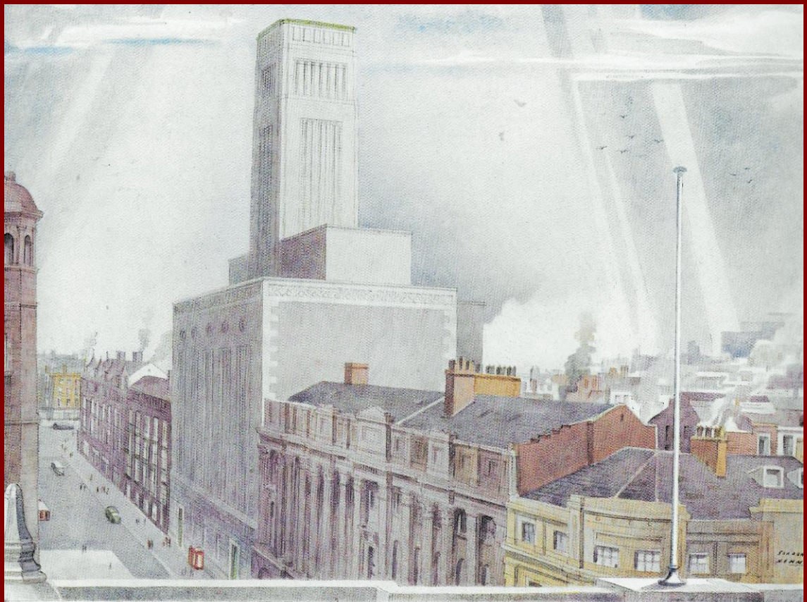
The Ventilation Station at North John Street, Liverpool
