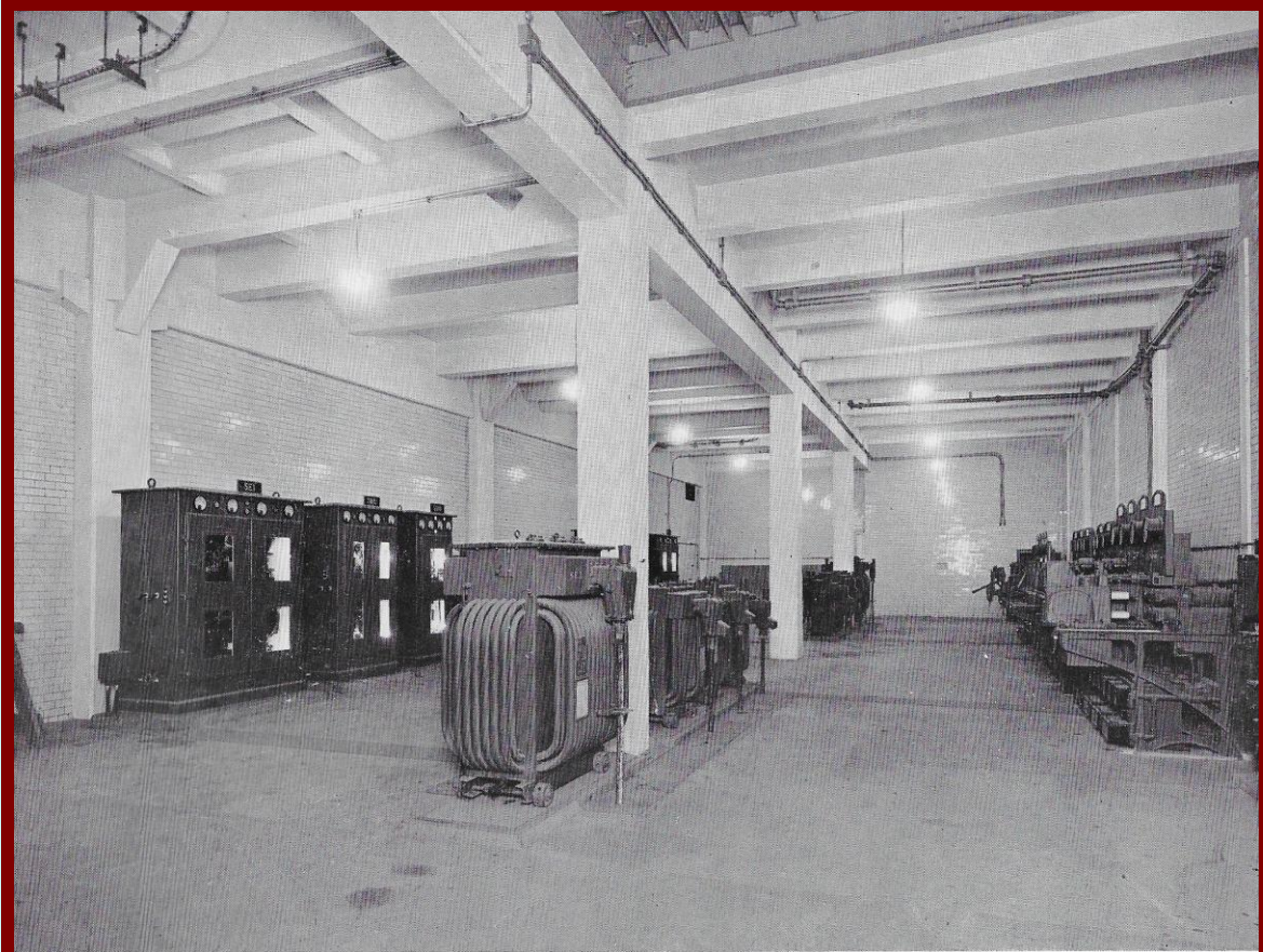
The switchgear room at Sidney Street ventilation station, Birkenhead
