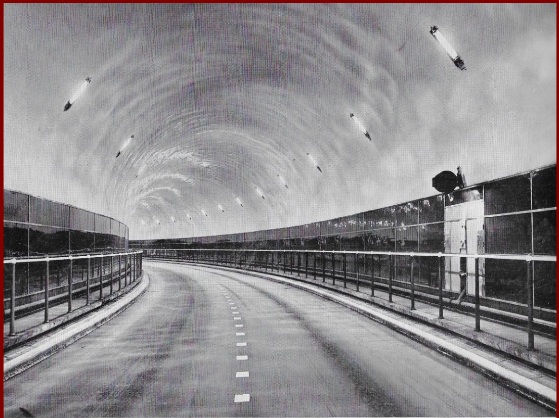
A curve in the branch tunnel
