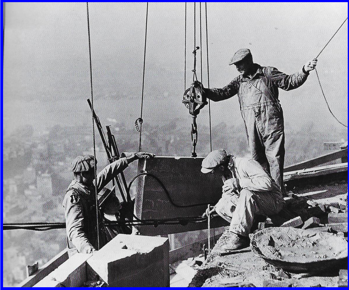
Lewis W. Hine photograph of Empire State Building stonemasons at work
