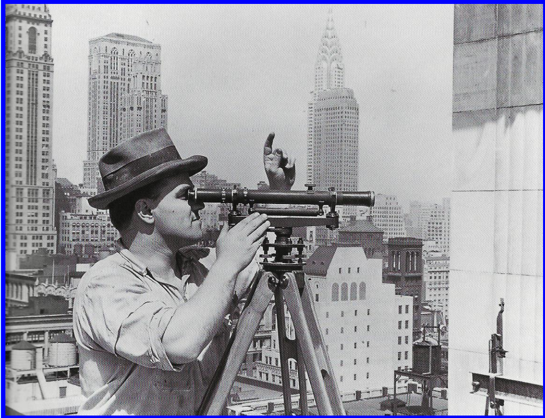
Lewis W. Hine photograph: Checking to see if the Empire State Building is "true"
