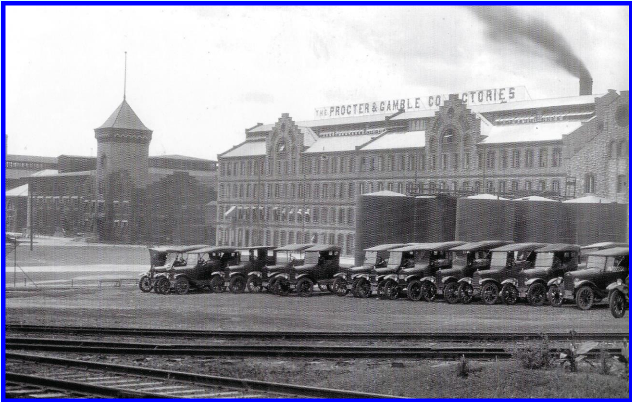
The Procter & Gamble Ivorydale, Cincinnati factory complex built 1886, photo 1927.
