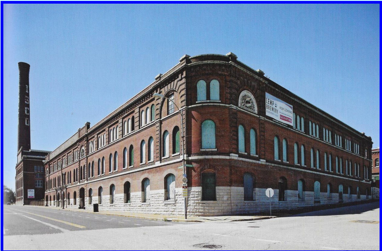
Once the largest brewer in St. Louis. Ruined by Prohibition, the complex is now used for storage.
