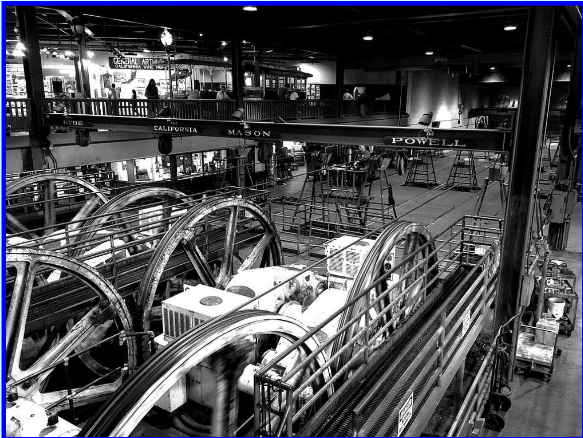
Two of the powerhouses and machinery once driving the historic cable car system.
