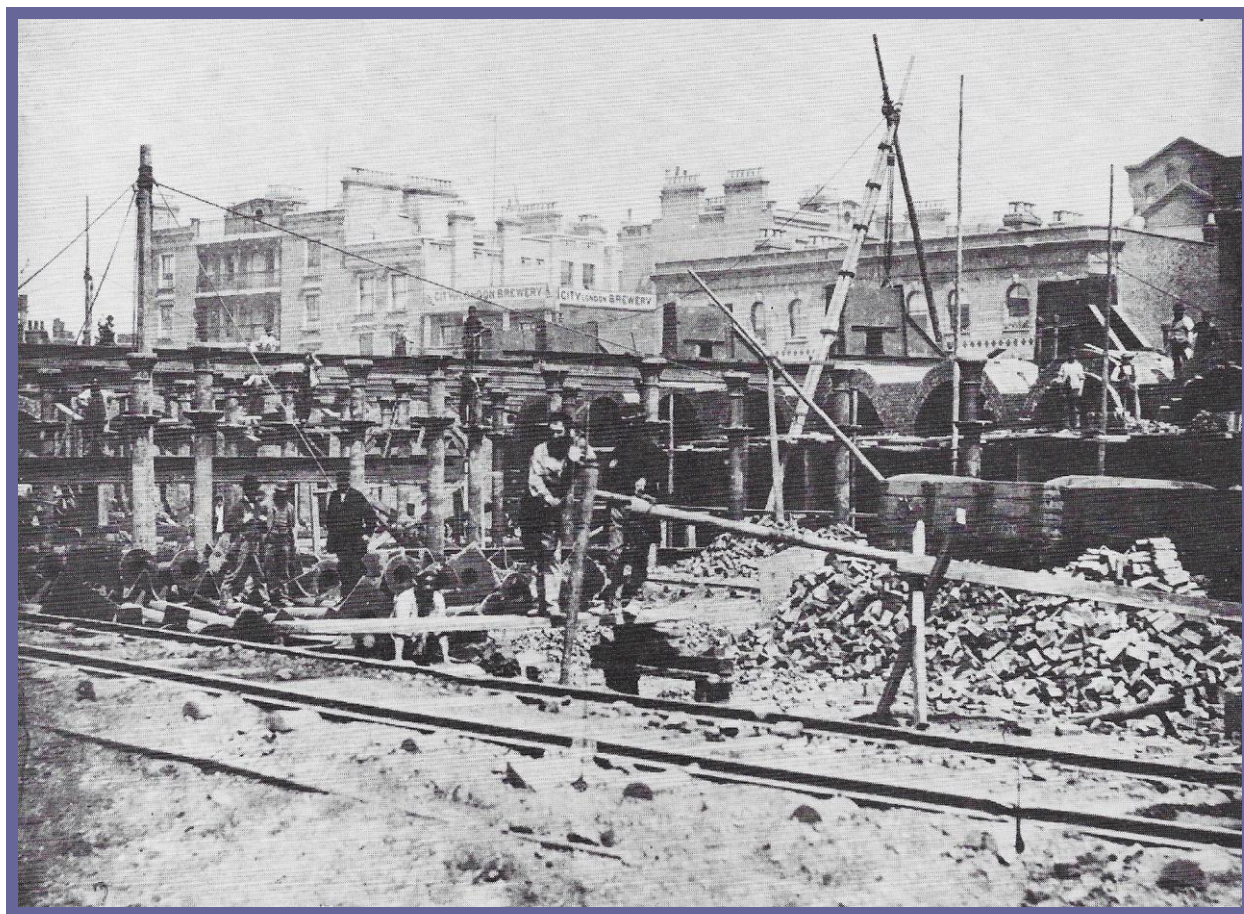
St. Pancras Station under construction c.1866-7.
