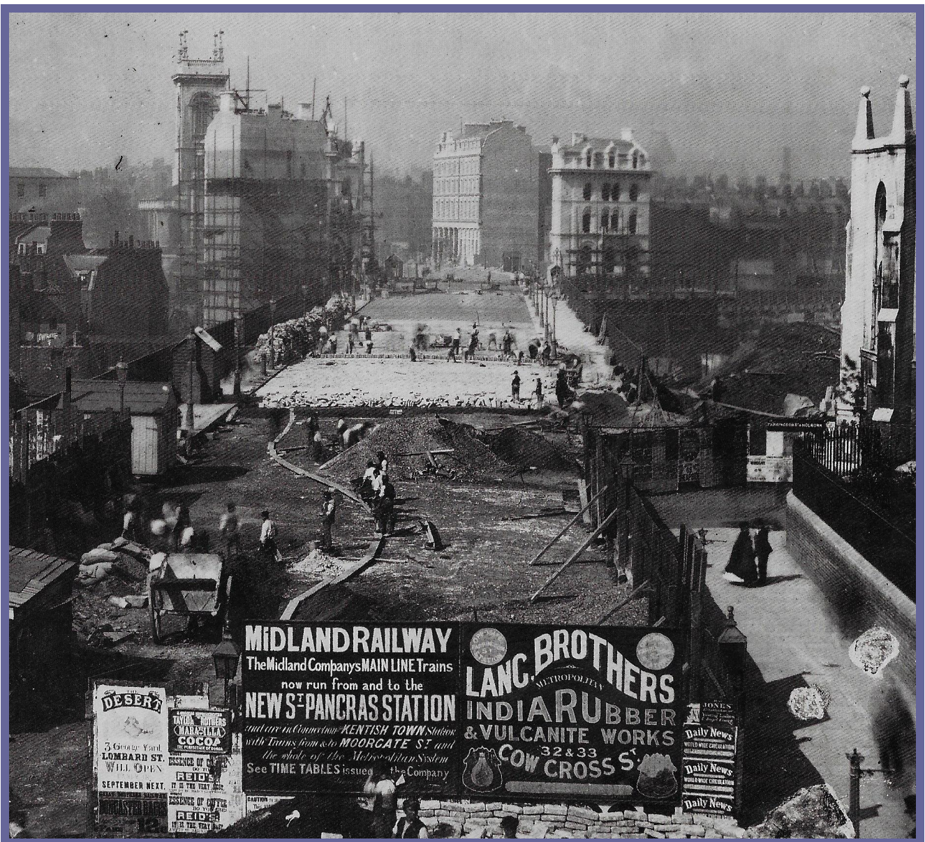
London's Holborn Viaduct under construction, 11 September 1869.
