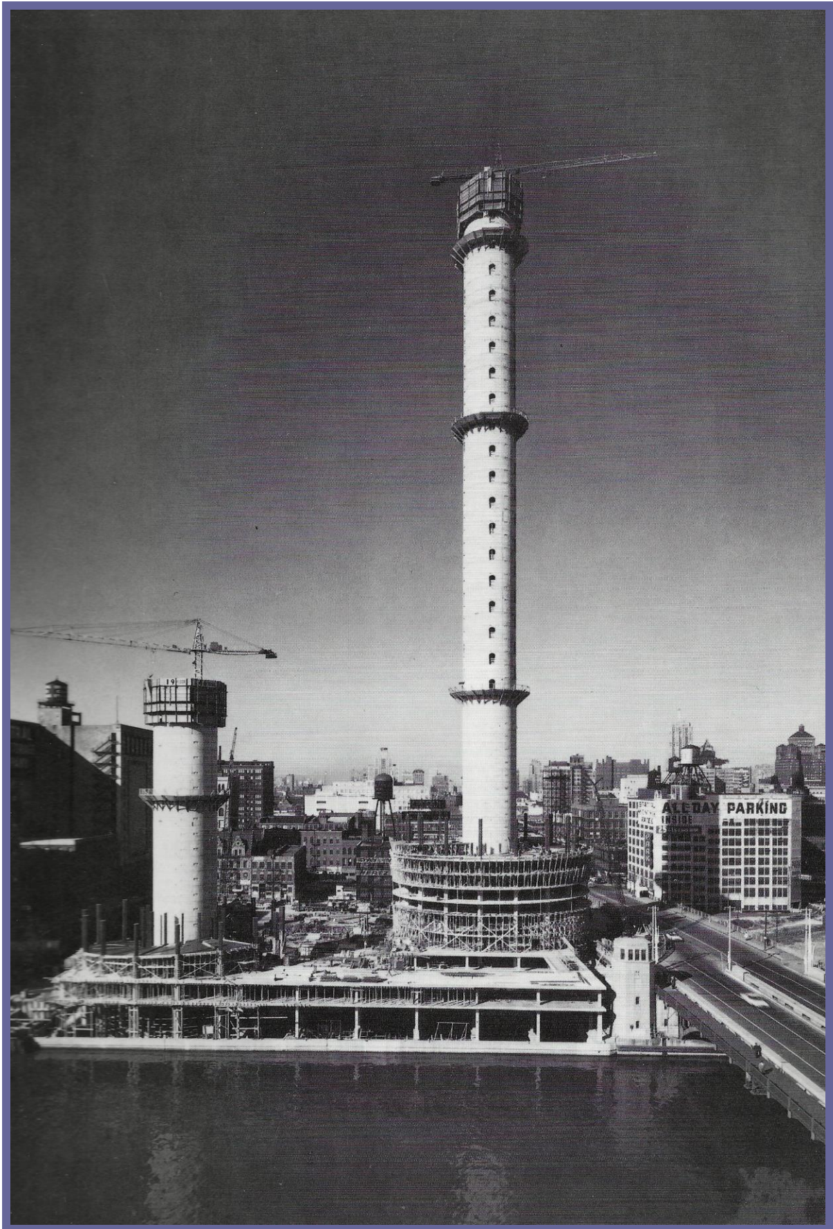
Built 1964. 588 ft high, 61 floors. Architect: Bertrand Goldberg. Lower 18 floors car parking. Upper floors apartments with individual heating and cooling units (no central plant).
