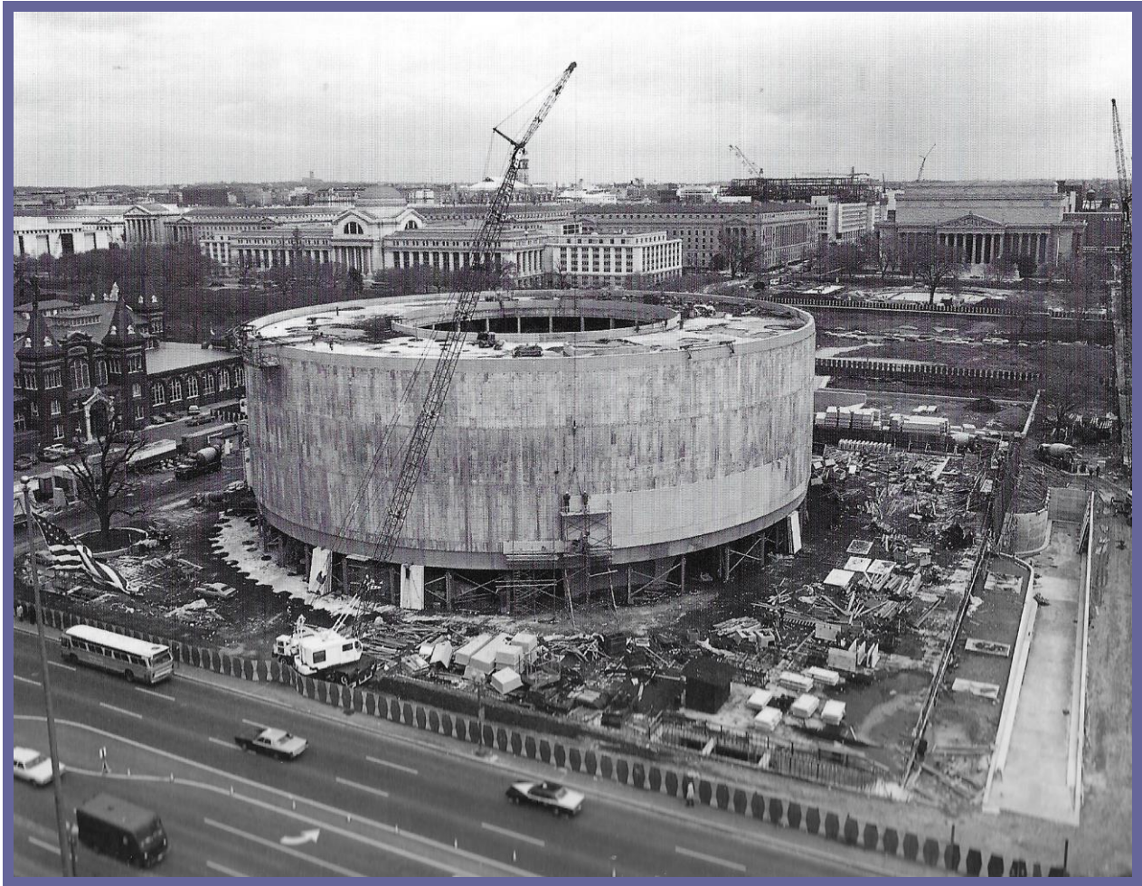
Constructing the Museum and Sculpture Garden on the Mall 1970-74. Architect: Skidmore, Owings and Merrill.
