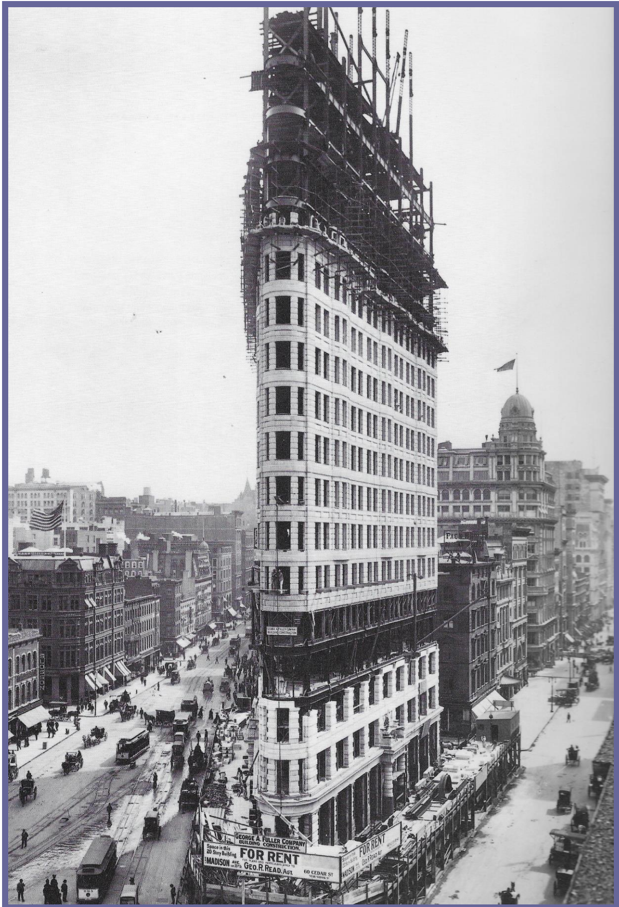
Built 1901-02. Architect Daniel H. Burnham. Real name was the Fuller Building, 300 ft tall. A steel-framed skyscraper clad in limestone.
