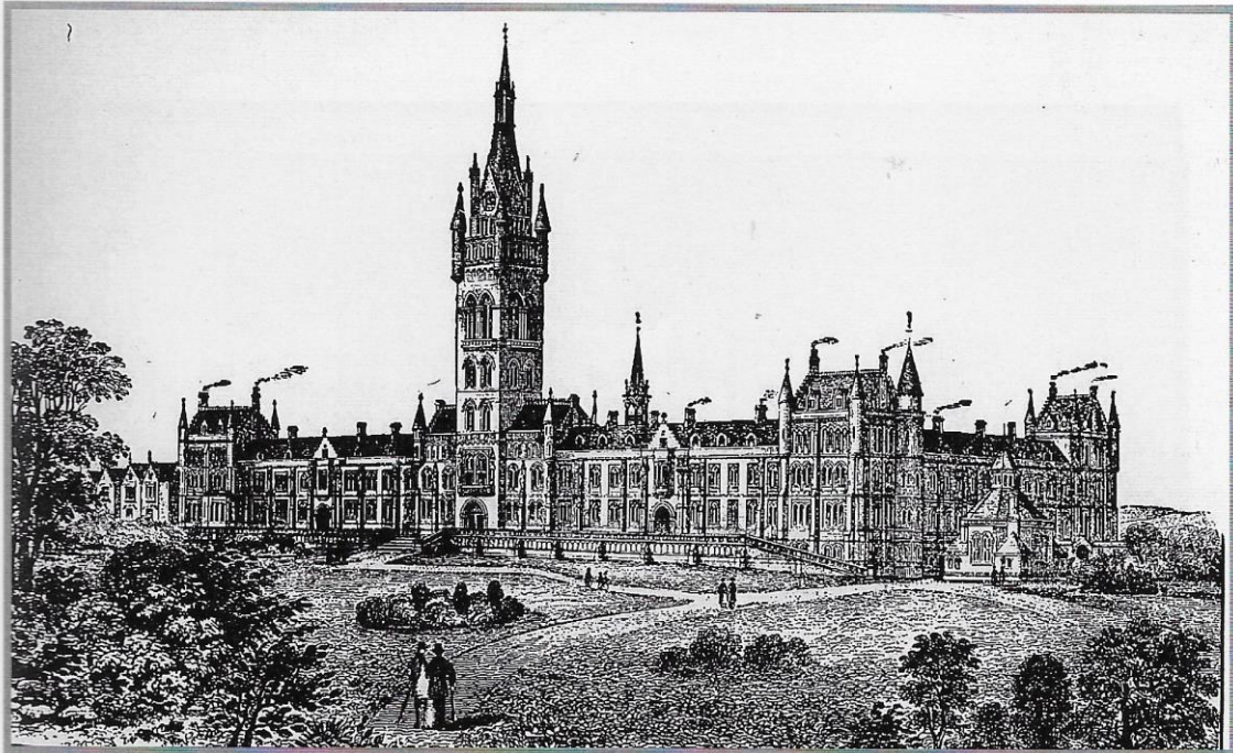
29. Sir G G Scott's Design for the University of Glasgow with his Proposed Tower (redesigned by his son, John Oldrid). Note the smoke from the heated exhaust ventilation shafts [MM, 135].
