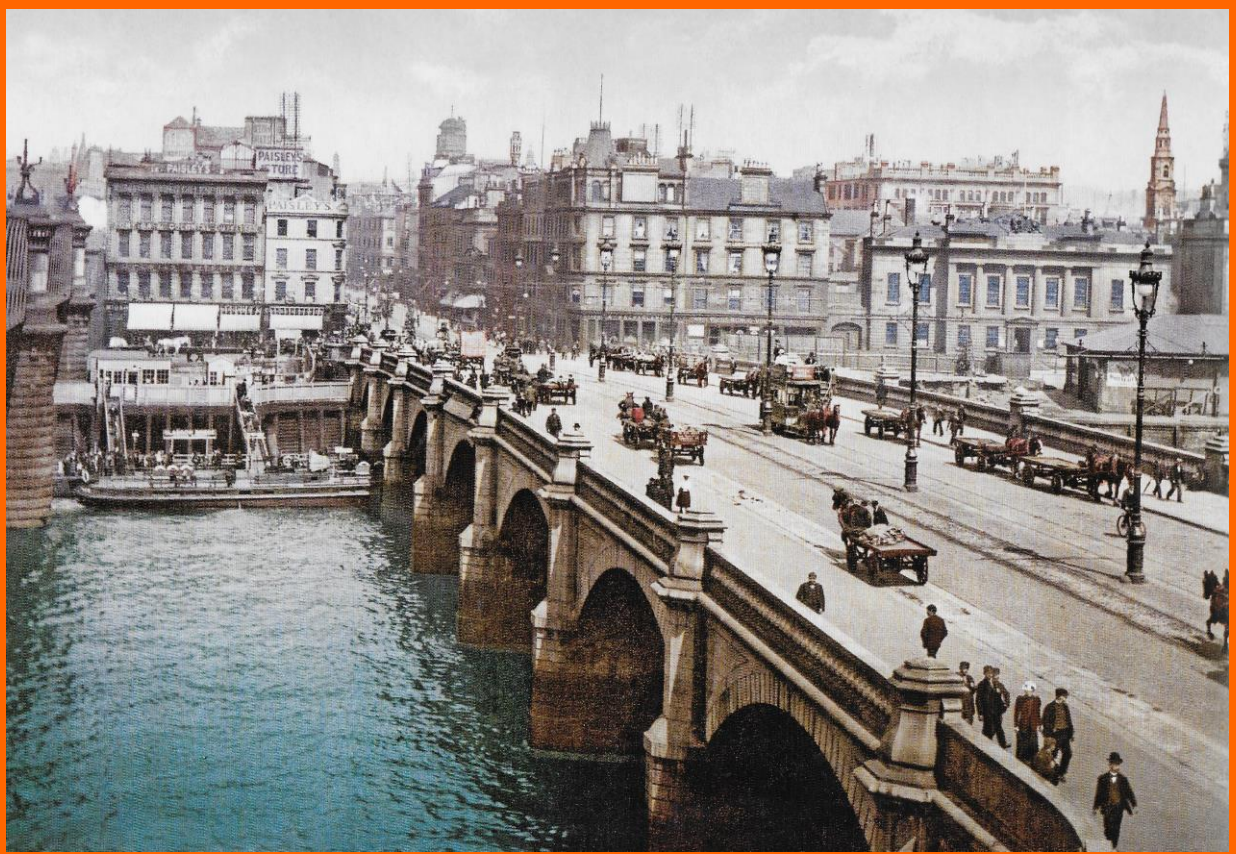
Glasgow Bridge, a hand-tinted photograph of 1910.
