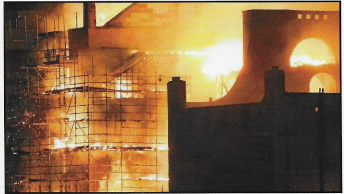
The Second Fire of 15 th June, 2018
