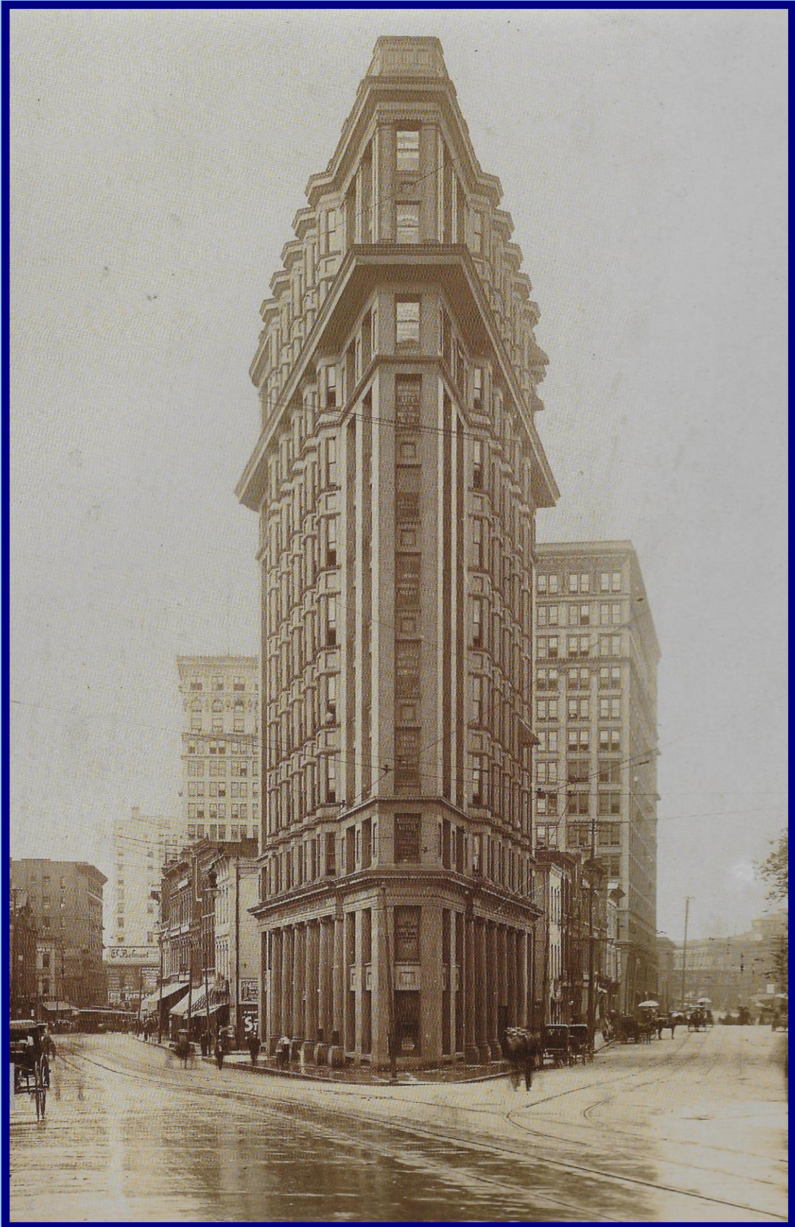
Photograph c.1900. Built 1897 as the English-American Building, Atlanta's oldest surviving skyscraper at 11 floors predates by five years New York's more famous Flatiron Building. Architect Bradford Gilbert.
