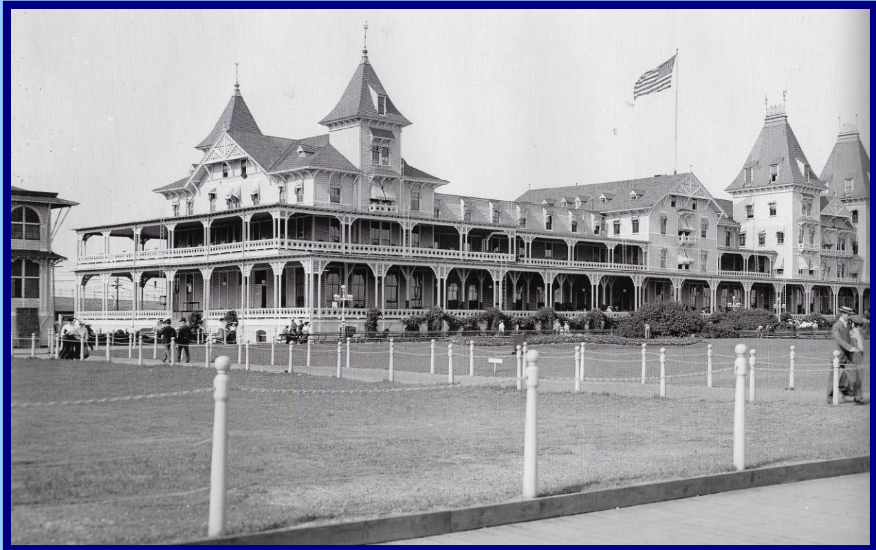
Photograph c.1910. Opened 1878. After the shoreline was damaged in blizzard of 1888, the 300 ft long building was jacked up, placed on 100 flatcars running on temporary rail tracks and moved from shore.
