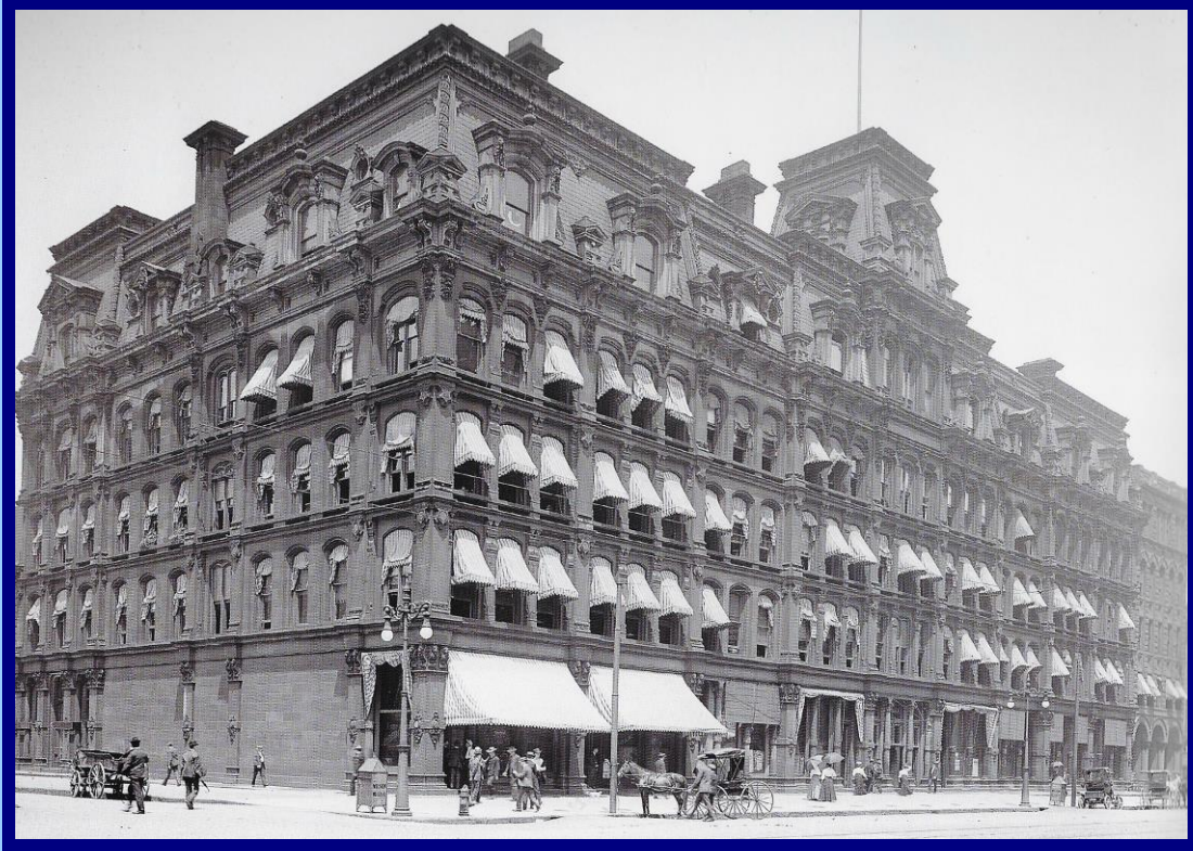
Opened 1875. Photograph c.1907. Changed from Club to City Hall to Public Library. Note the external (sunshade) awnings at windows in days before air conditioning.
