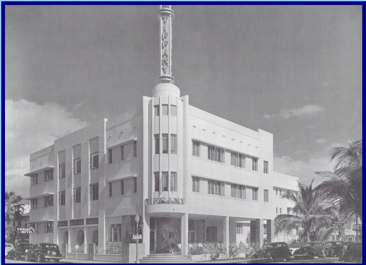
Photograph and built 1939 in Art Deco style. Architect L. Murray Dixon.
