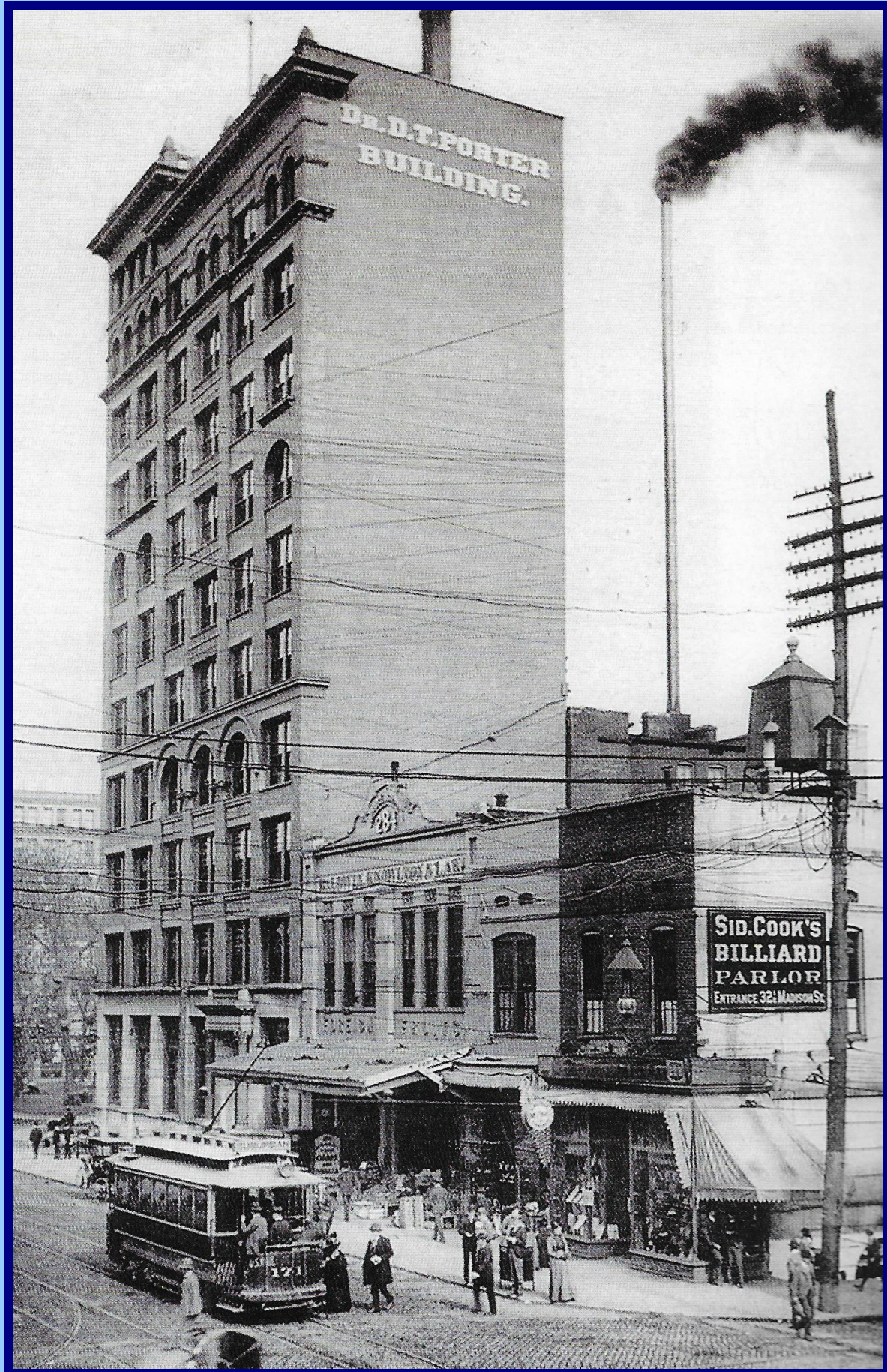
Photograph 1900. Built 1895 with 11 floors plus penthouse and basement. Claimed the first "circulated-water heating system" and city's first elevator.
