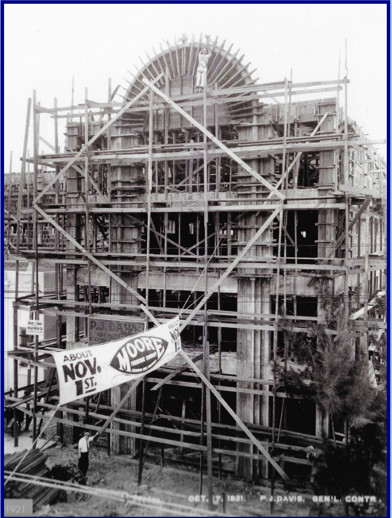
Photograph under construction 1921. Buena Vista was incorporated into Miami in 1924.
