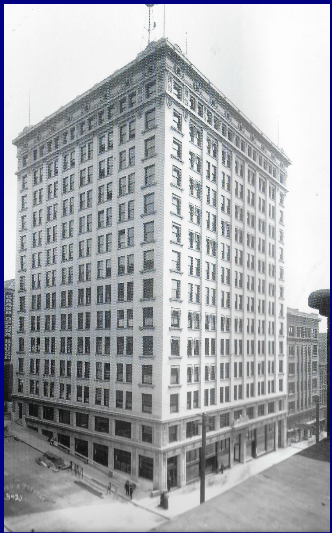
1903 photograph of Seattle's first skyscraper with steel framing, 14 floors.
