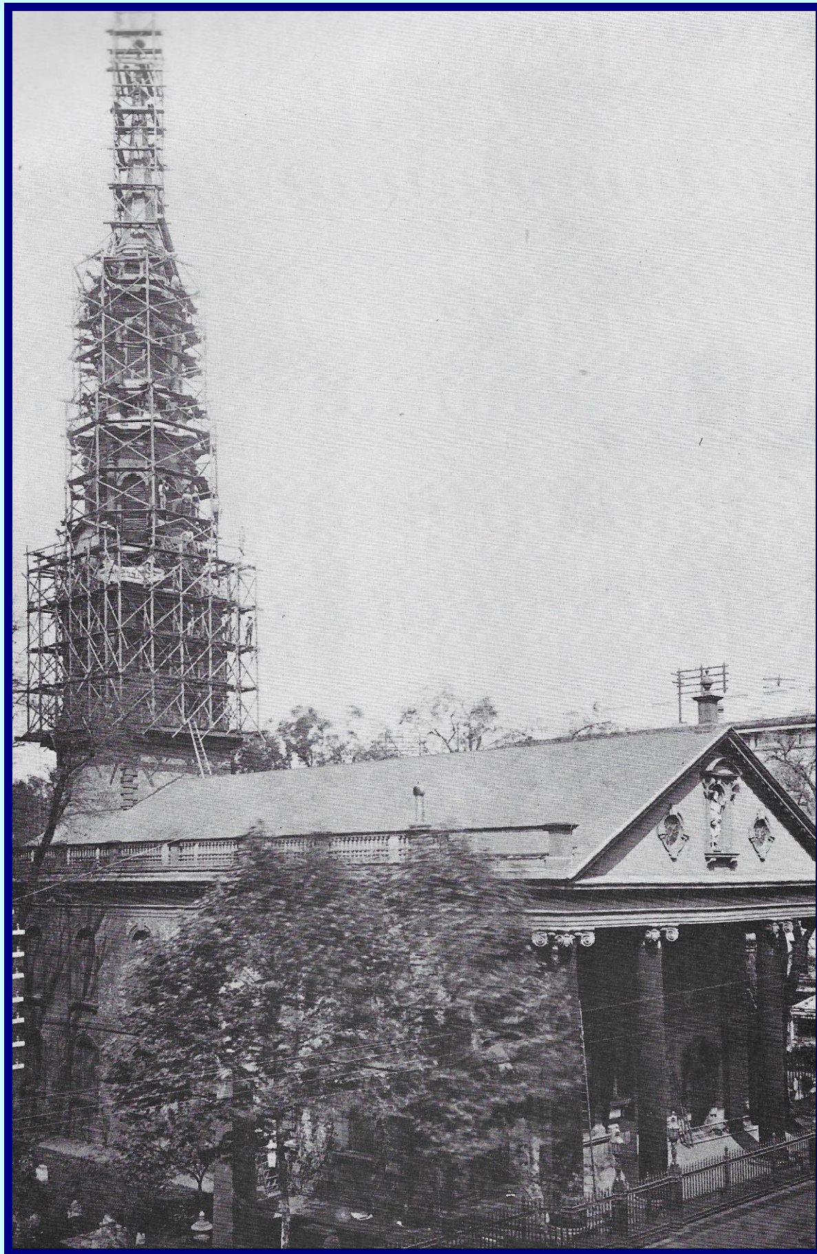
Photograph of 1881 shows repairs underway to the Chapel steeple of 1796.
