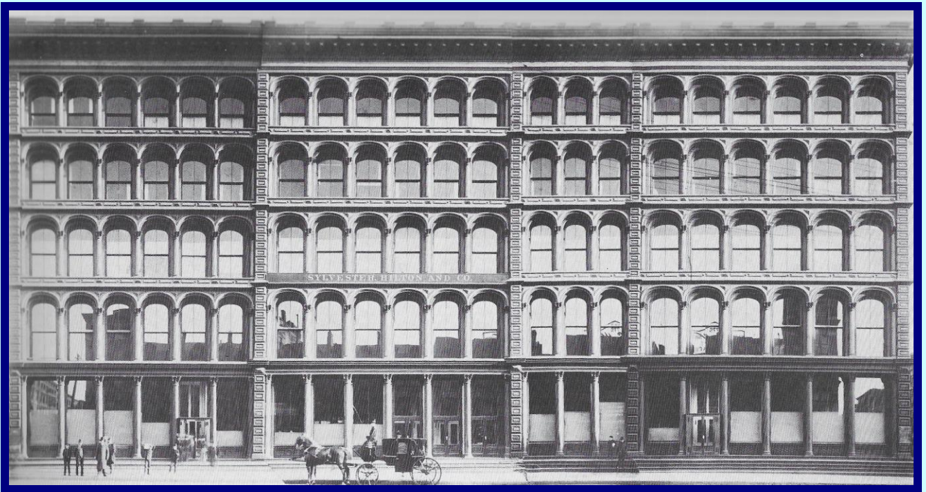
East Side of Broadway c.1885. Composite View (Three Photographs) of Department Store Block. Neo-Venetian style cast-iron building.
