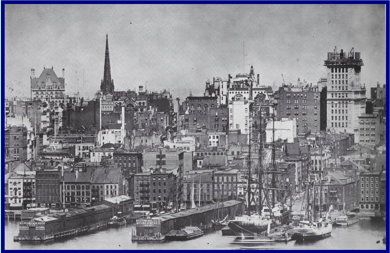
East River Piers 1888.
