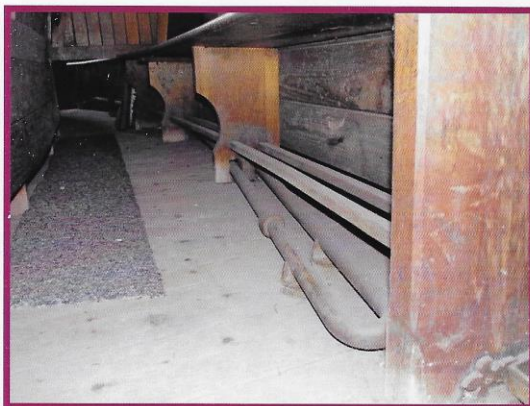
The low-level MPHWH Perkins pipework heating coils
