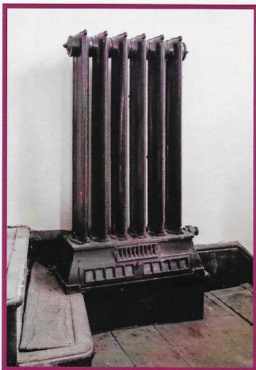
Examples of the flueless direct-fired gas radiators
