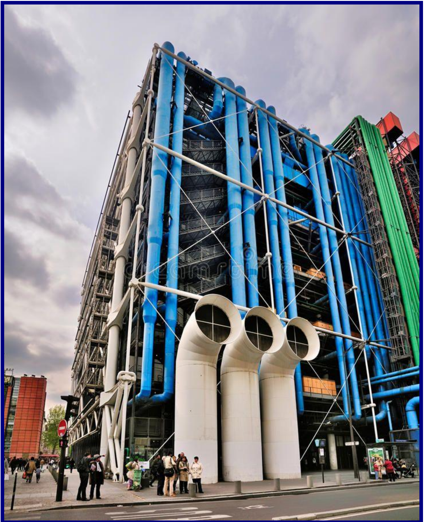
Example of the colour coding of external services.
