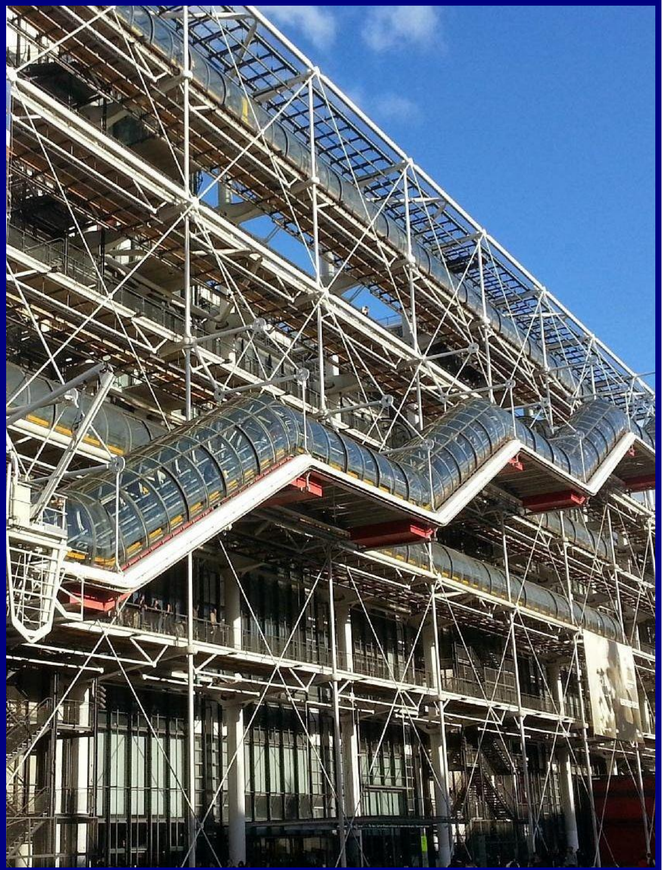
The external "stepped" escalator within a tube.
