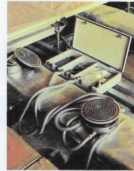
Underfloor air distribution system (1985)
