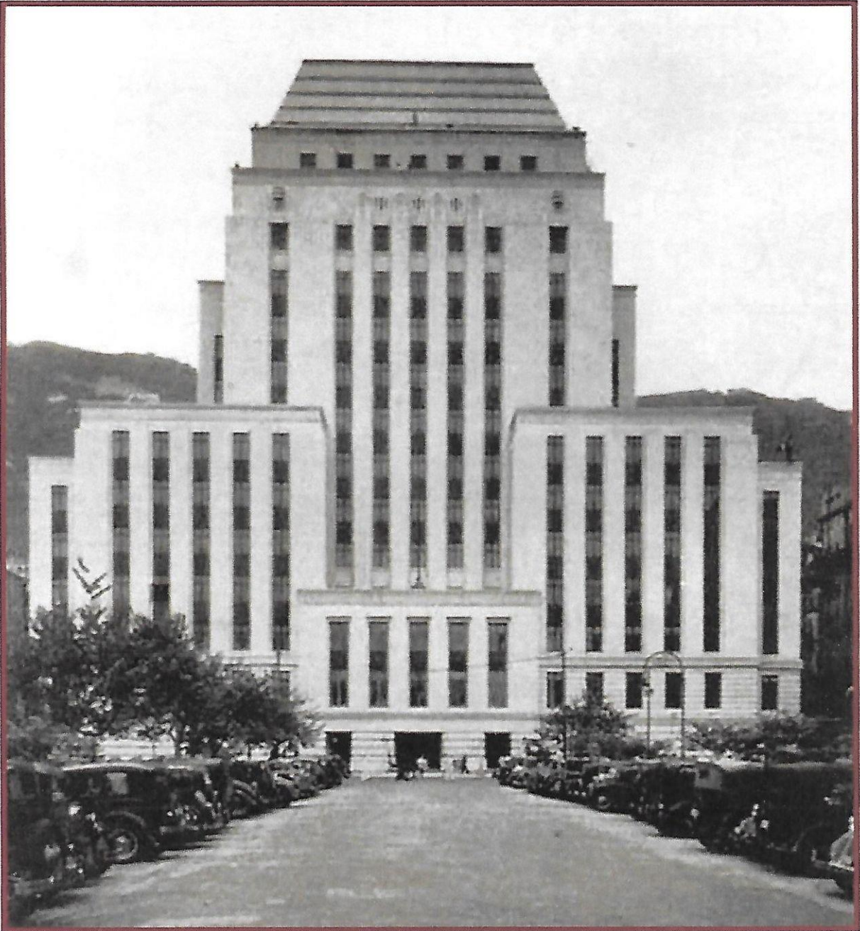
1936 The Hongkong & Shanghai Banking Corporation, New Head Office, Hong Kong Air conditioned by G N Haden & Sons Ltd who provided ammonia refrigerating machines (410 hp) serving six air handling plants (229,000 cu.ft/min supply air), contract value being £75,000
