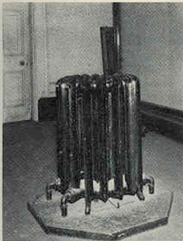
Purpose made "column" radiator at the V & A Museum (c. 1900)
