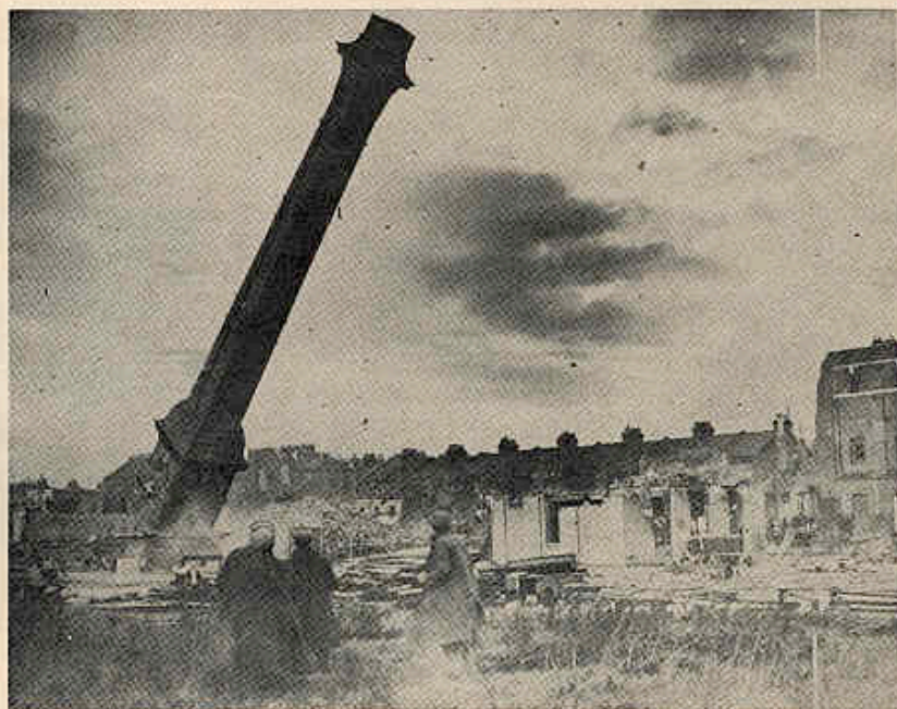
Demolition of an old chimney by Beaumonts in the 20's
