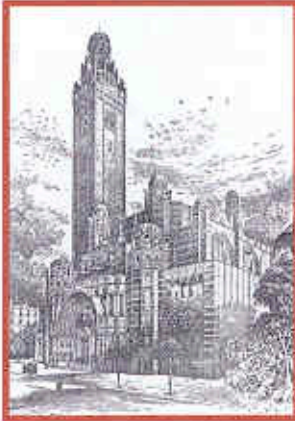
1927 Westminster Cathedral (Boilers converted to oil-firing by G N Haden & Sons)
