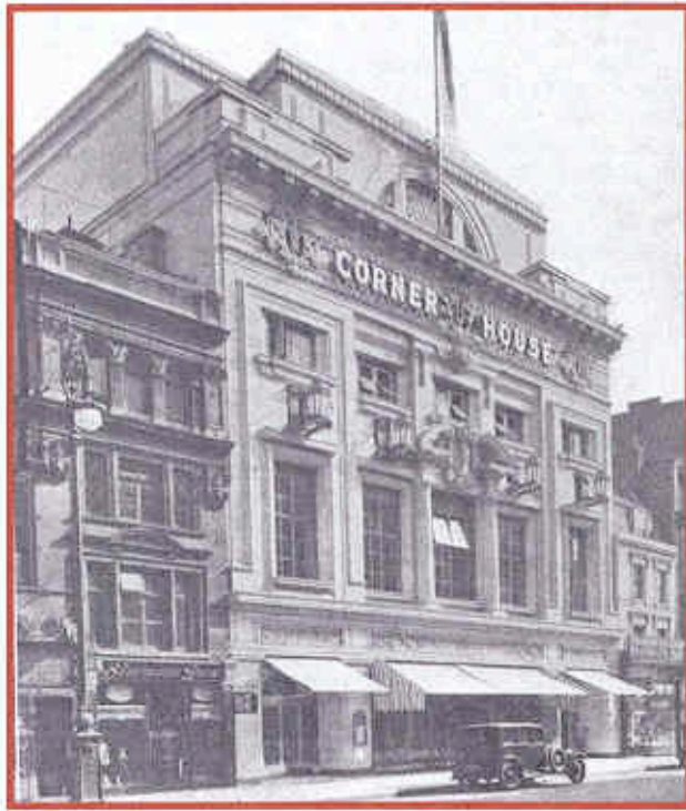
1928 Corner House, Oxford Street (Heating by J Jeffreys)
