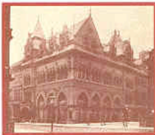
1904 Stock Exchange, Glasgow (LPHW heating using Reck steam accelerator by James Boyd)
