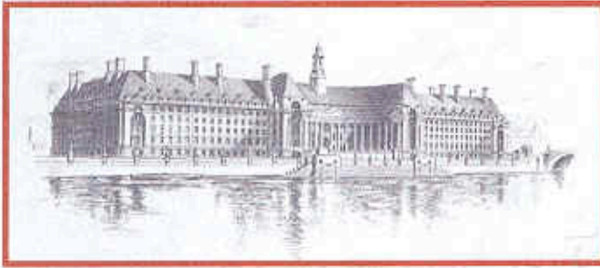
1922 London County Hall (Heating and ventilation by a consortium of Jeffrey's, Crittall, Haden, Norris & Dutton)
