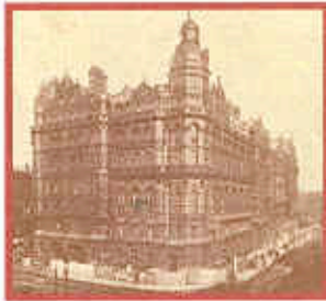
1903 Midland Hotel, Manchester (Heating by Ashwell & Nesbit)
