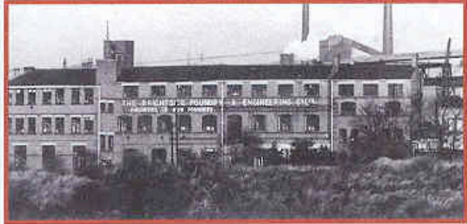
Brightside Foundry, Sheffield
