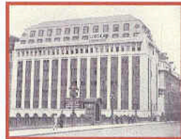
1929 Vintry House, Queen Street Place, London (Heating by J Jeffreys)
