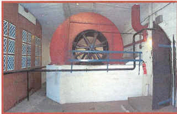
1911 Central Methodist Hall, London (Heating and ventilation by Ashwell & Nesbit)
