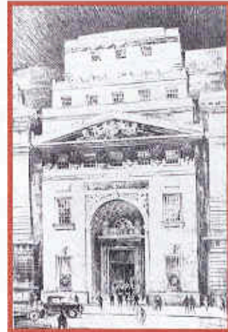
1928 Lloyds HQ, London (Heating and ventilation by Mumford Bailey & Preston)
