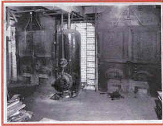
(Boiler plant by Ashwell & Nesbit) 1911 Central Methodist Hall, London
