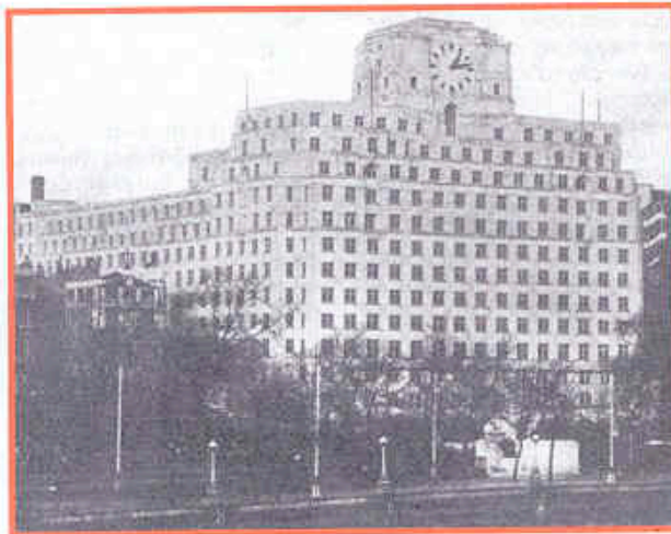
1934 Shellmex House, Thames Embankment, London (Under-window concealed radiant panels by Young, Austen & Young)
