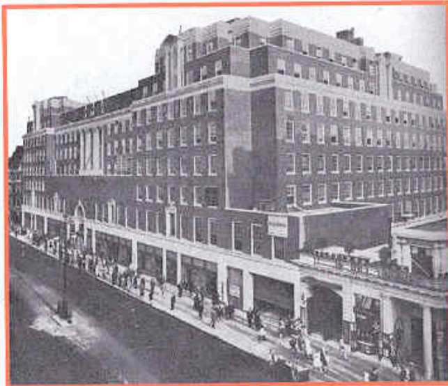
1930 Gamage's Department Store, Oxford Street, London (Heating by G N Haden & Sons)
