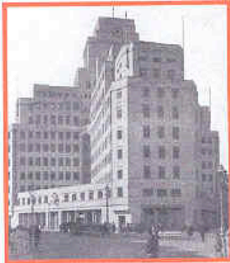
1930 London Transport 55 Broadway, London SW1 (Electric thermal storage heating by Richard Crittall)
