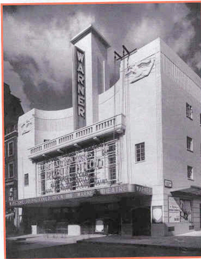
1938 Warner Theatre, Leicester Square, London (Air conditioning by Carrier Engineering)
