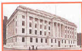
1932 Wellcome Research, London (Heating and ventilation by G N Haden & Sons)
