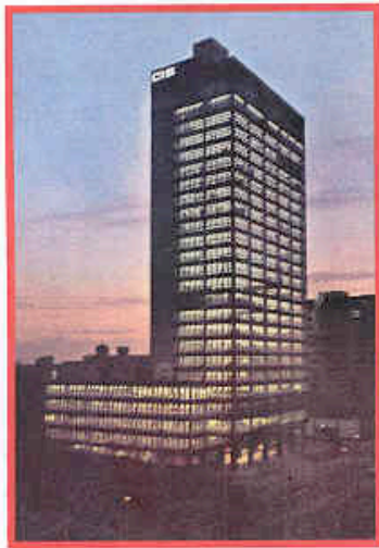
1962 CIS, Manchester (Air conditioning, Carrier Engineering)
