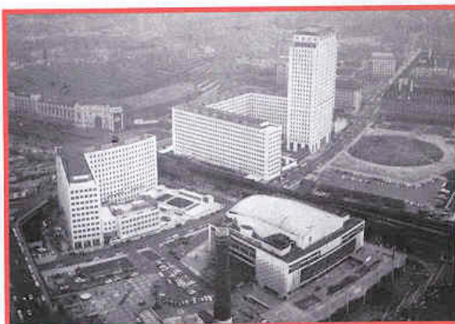
1962 Shell Centre, South Bank, London (Air conditioning by chilled radiant ceilings, G N Haden & Sons)
