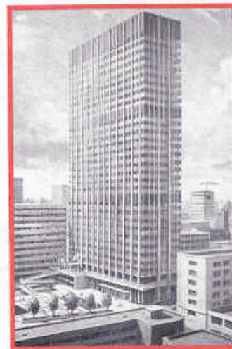
1967 BP Moorfields, London (Air conditioning by Brightside)
