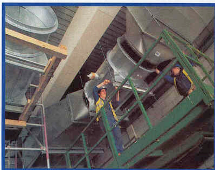
Ductwork manufacture and erection (Richard Irvin)
