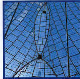
Perspex roof, Olympic Stadium, Munich. Günter Behnisch & Frei Otto, 1972
