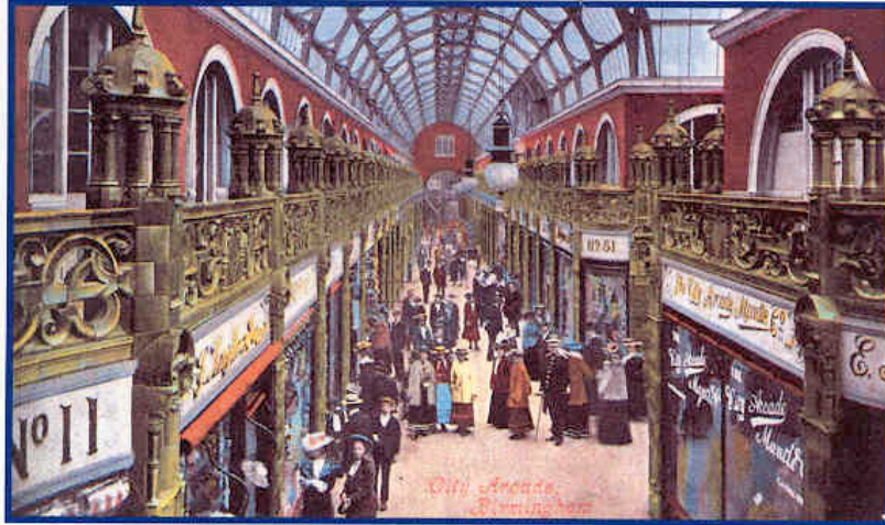
The Great Western (City) Arcade, Corporation Street to Colmore Row, Birmingham, built 1902. [The Story of Typhoo, Ken Williams, 1990]
