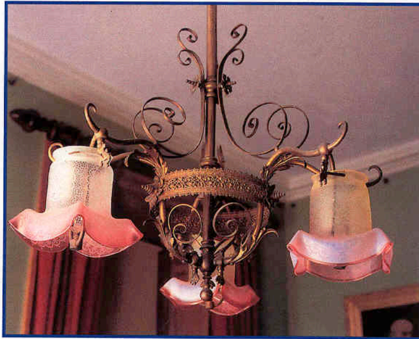
Ornate three- arm gasolier, originally for acetylene at The Argory, County Armagh. Designed to have the appearance of an electrolier, possibly made by The Welsbach Incandescent Gas Light Company. [Artificial Sunshine, Maureen Dillon, The National Trust, 2002]
